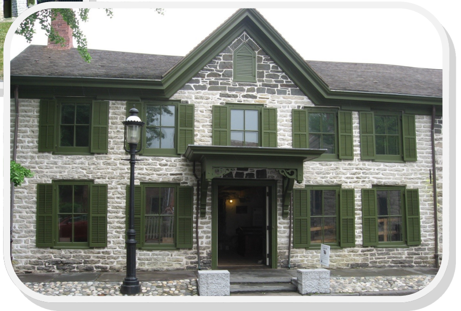
Phase 4 (John Street)
