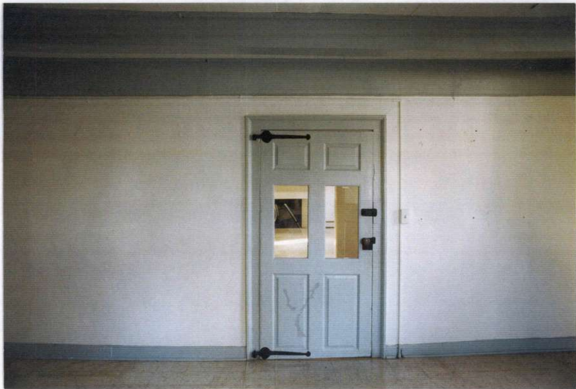
53. Space 101 south wall. Door with Dutch strap and pintel hardware.
