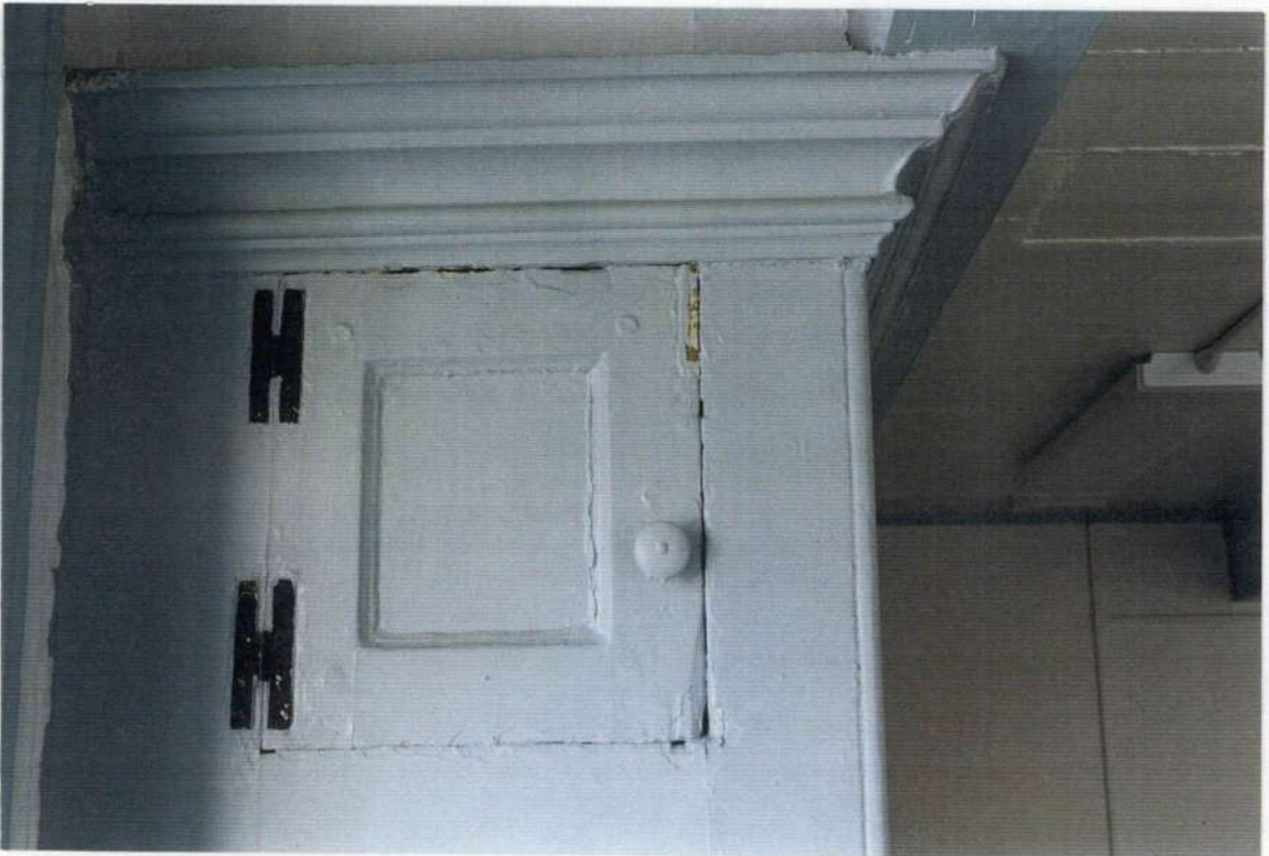
47. Space 101. Detail of warming cupboard at west end above fireplace mantel.
