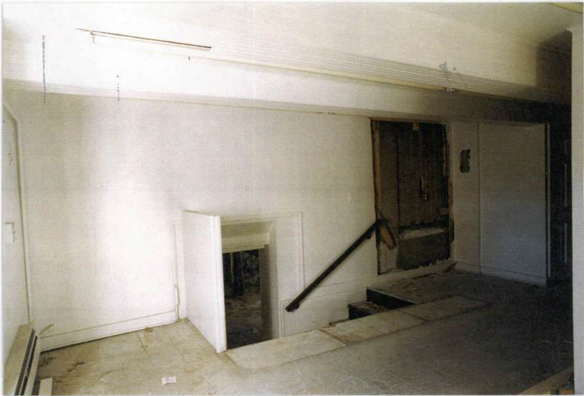
134. Space 104 west wall before removals.
