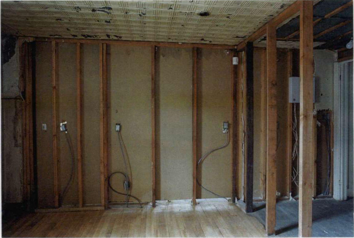
232. Space 112 south wall before removals.
