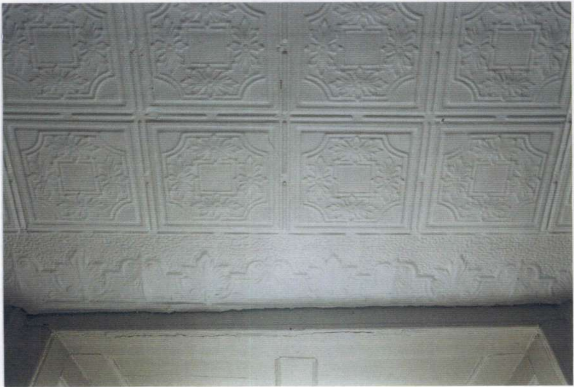
113. Detail: Tin ceiling of space 103.
