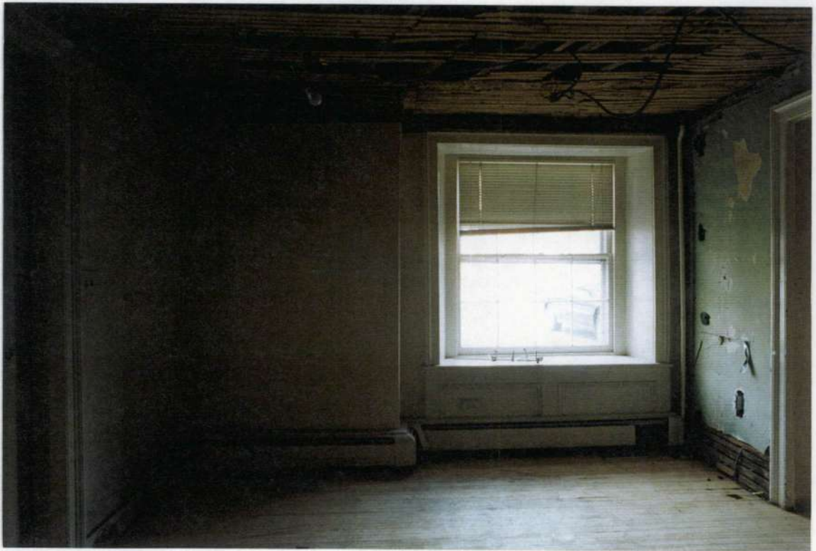
190. Space 109 east wall after removals. Note blocked in fireplace.
