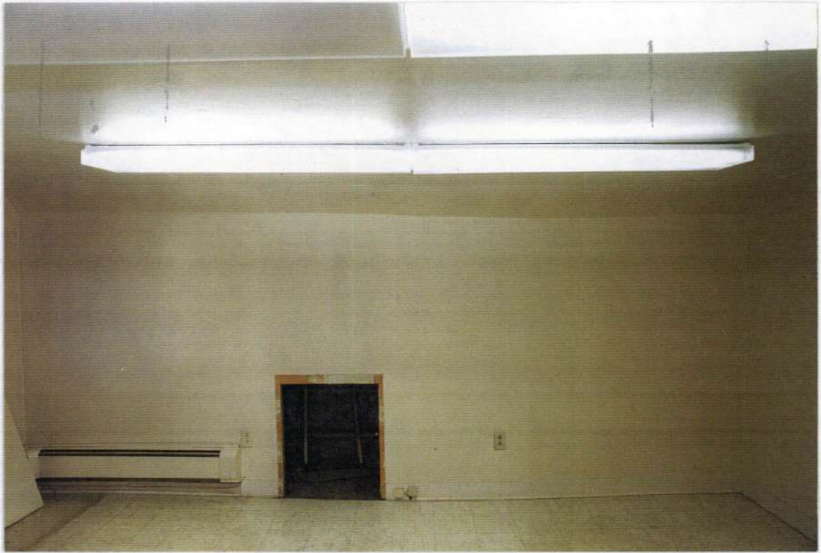
120. Space 204. West wall before removals.
