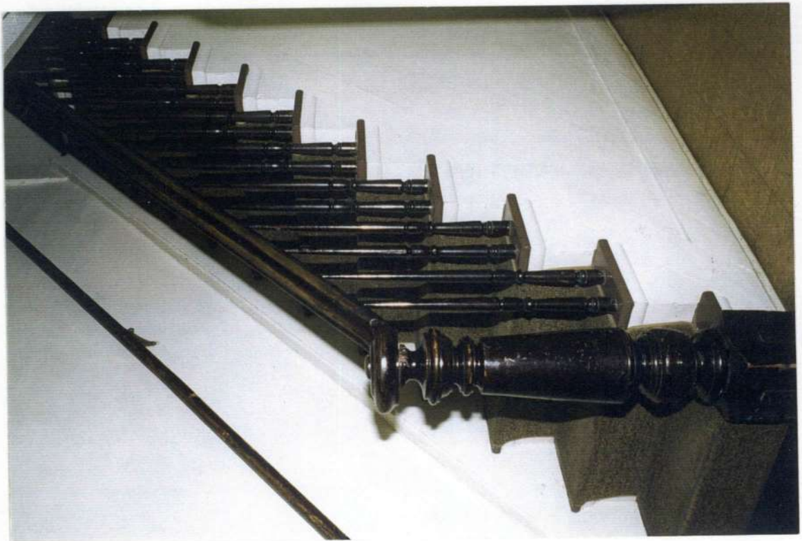
161a. Space 107 stair hall. Stair and railing.
