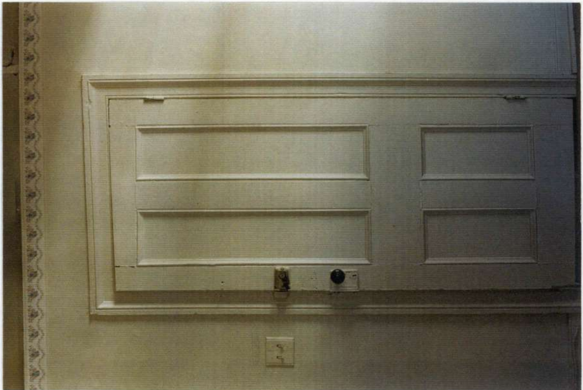
214. Door between space 206 and 207 as seen from 207.
