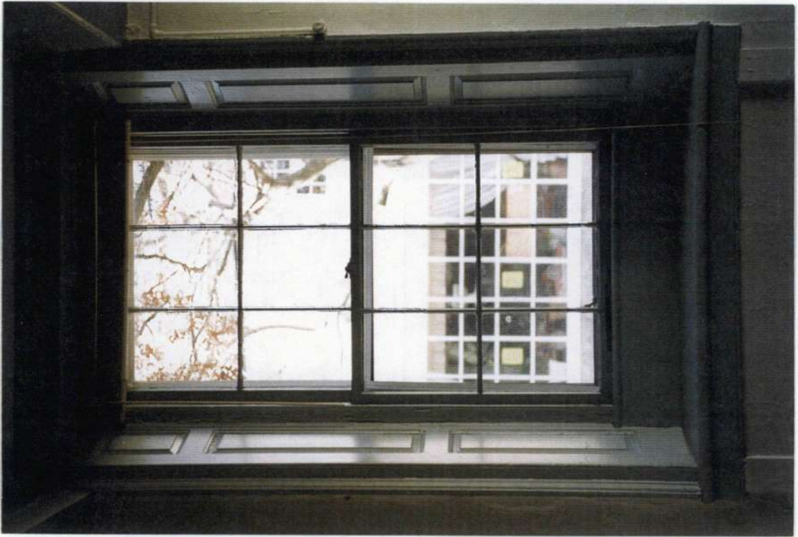
50. Space 101. West wall raised panel detailing of wood window surround.
