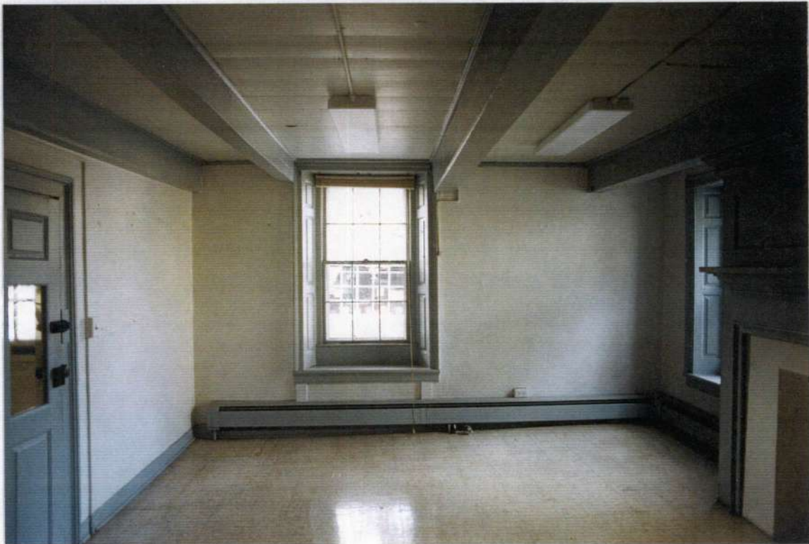
45. Space 101 west wall. Paneled window, beam ceiling with exposed wood planks. Note smaller beam to left of window. May be replacement beam.
