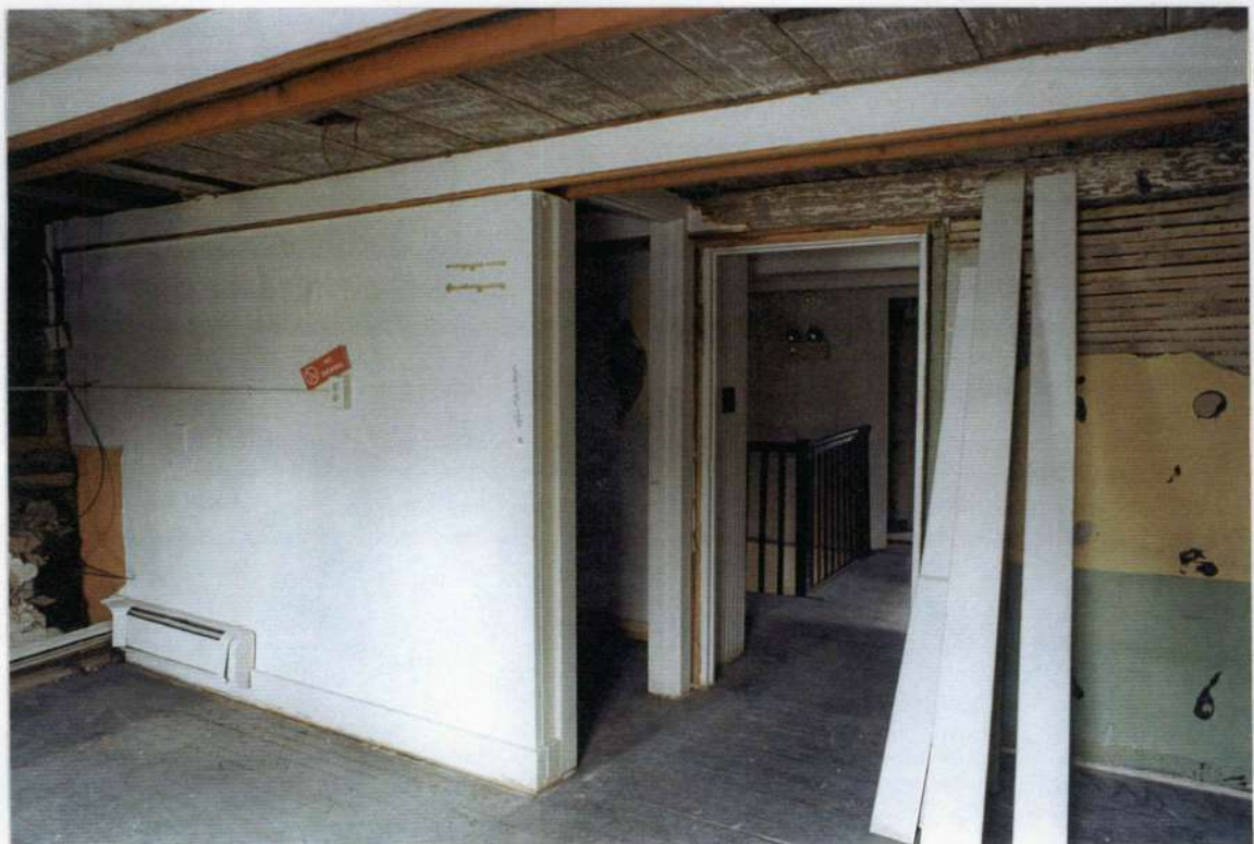
84. Space 201. South wall after removals.
