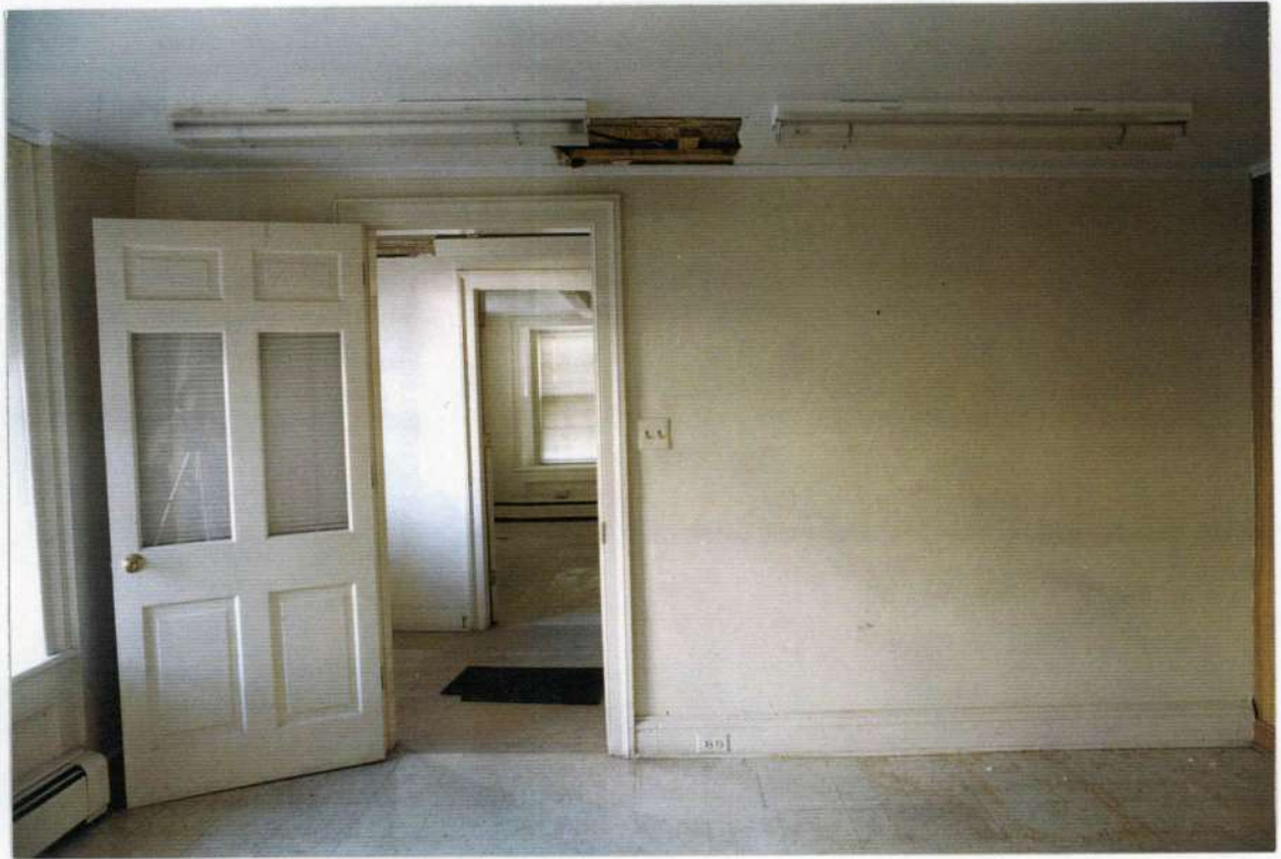
168. Space 105 east wall before removals.
