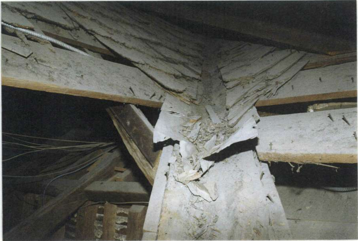
152c. Abandoned valley gutter intersection of phase two and three roofs.
