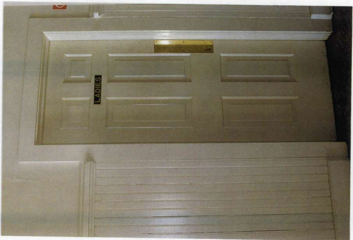
229a. Door to space 110B with wainscoting wall.
