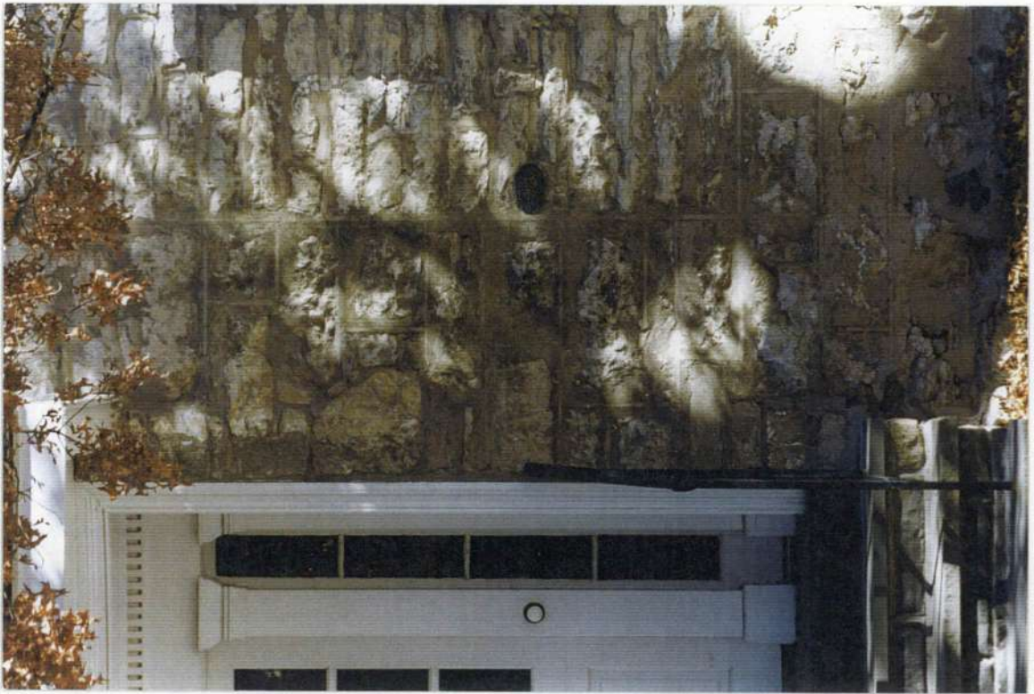
20. Joint in stonework between phase one and phase two.
