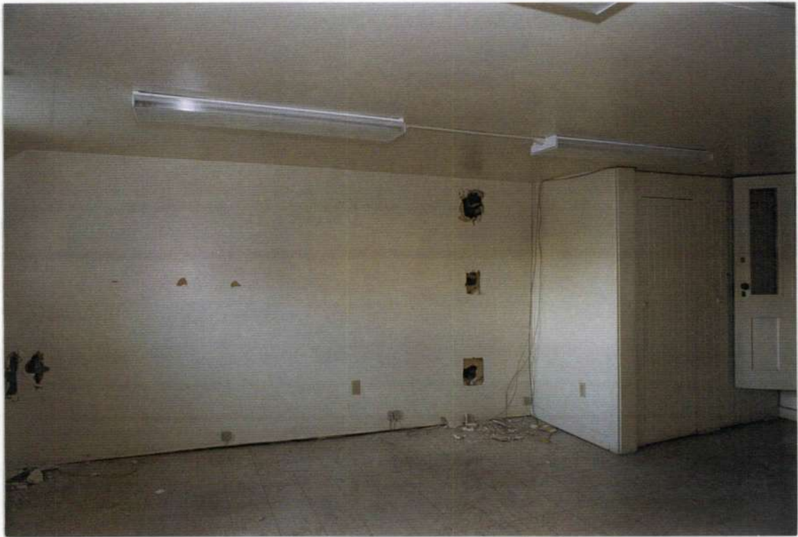
142. Space 205. West wall before removals.
