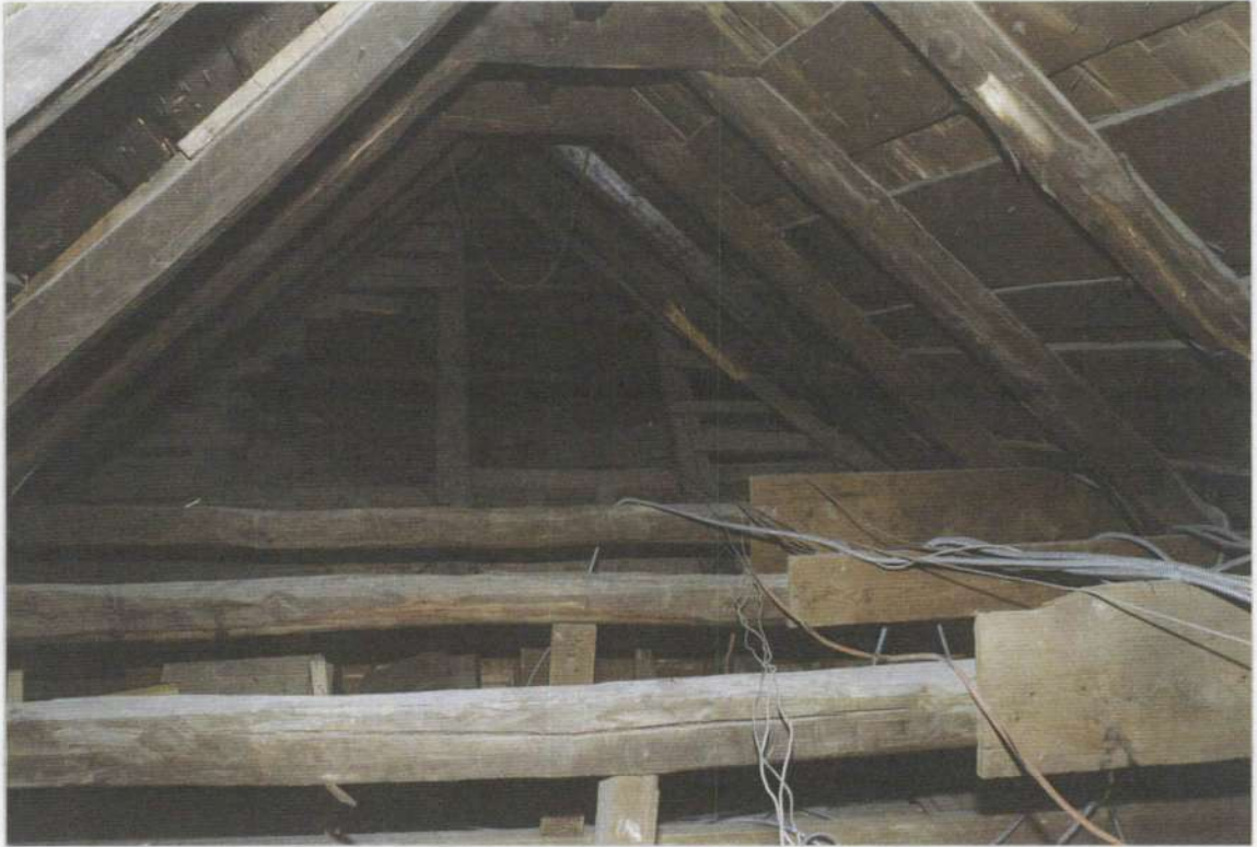
148u. Attic over space 205 looking west toward phase two roof.
