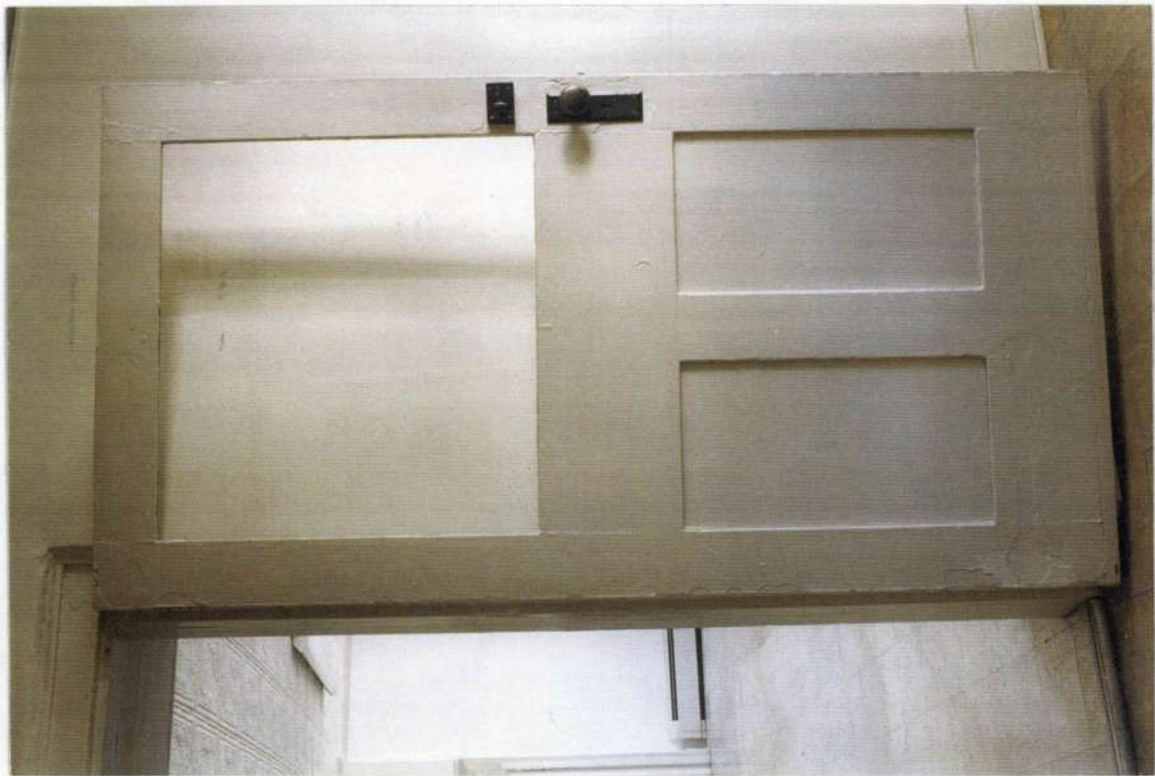
111. Detail: Space 103 side of door. Note shadows of Dutch pancake style strap hinge top and bottom. This door swing was reversed. The frame has pintel holes where door was hung on hall side of frame.
