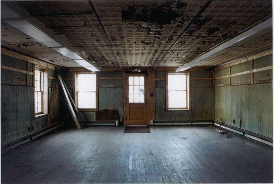
234. Space 113 south wall after removals.
