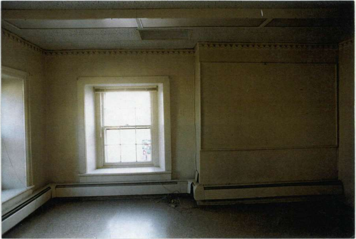
205. Space 207 east wall before removals. Note blocked in fireplace.
