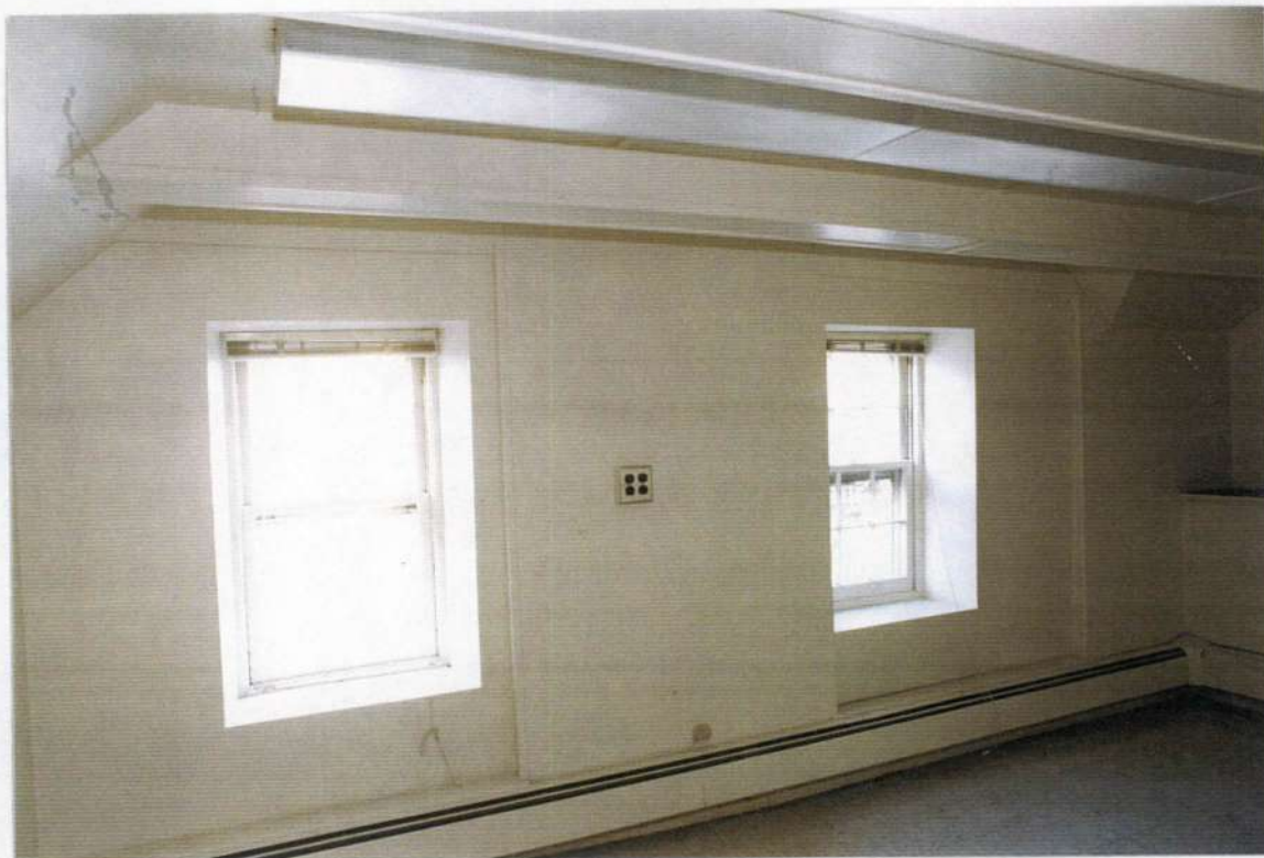
71. Space 201. North wall before removals.
