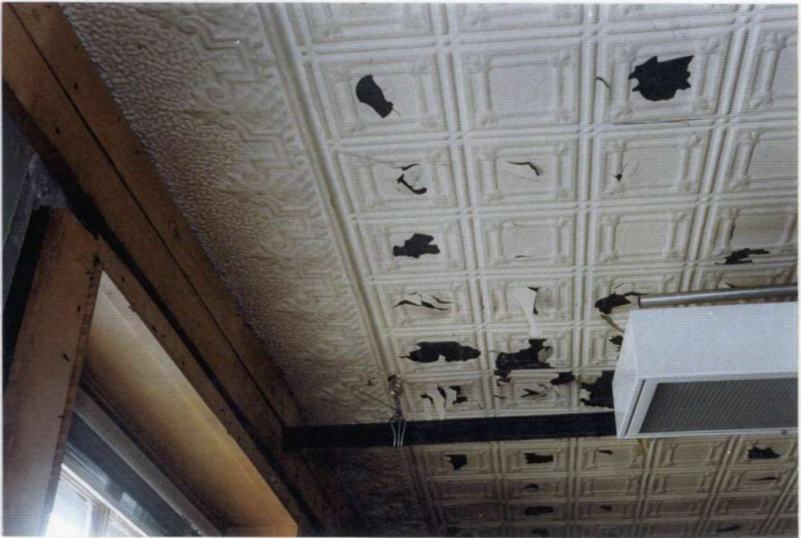
233. Space 112 and 113 tin ceiling after removals.
