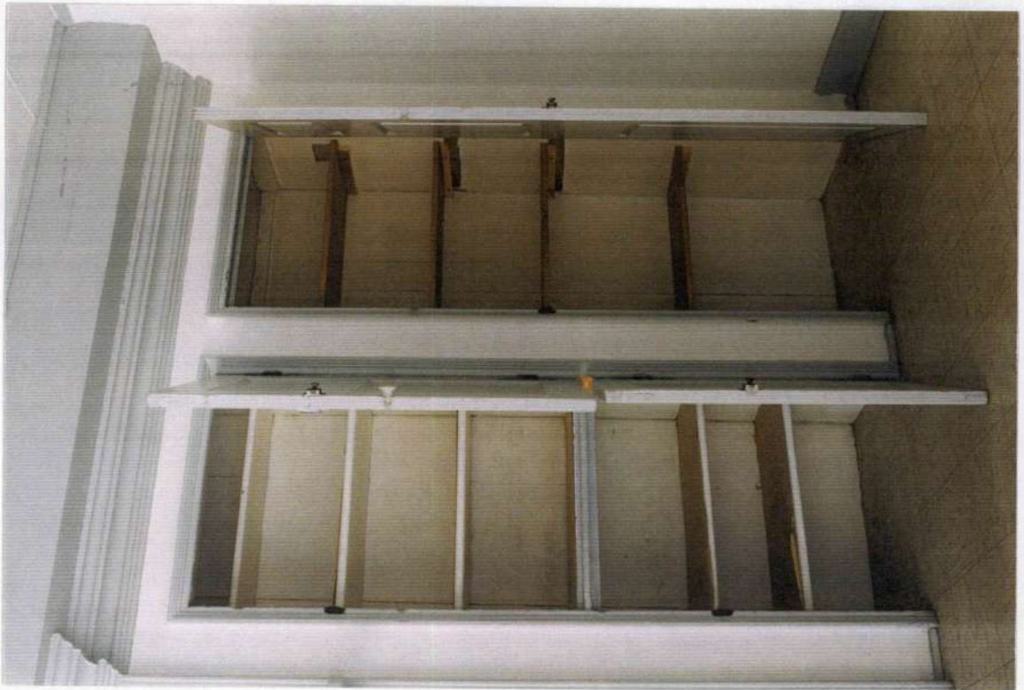
49. Exterior of fireplace cupboards: flat panel detailing. Doors have raised panel detailing on interior side.
