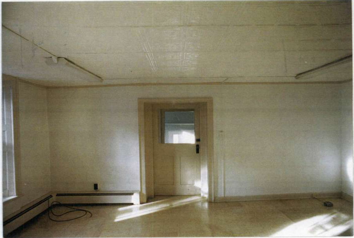
108. Space 103 North wall
