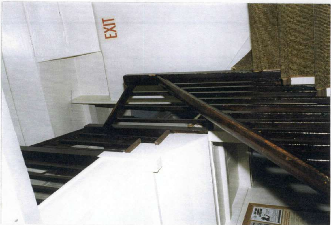
57. Detail: Stair railing and ceiling beyond.
