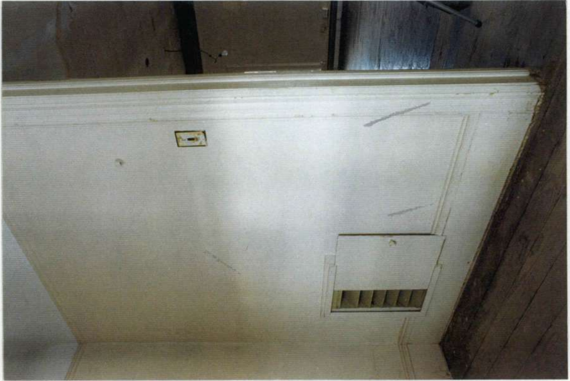
252. Space 214 east wall after removals.
