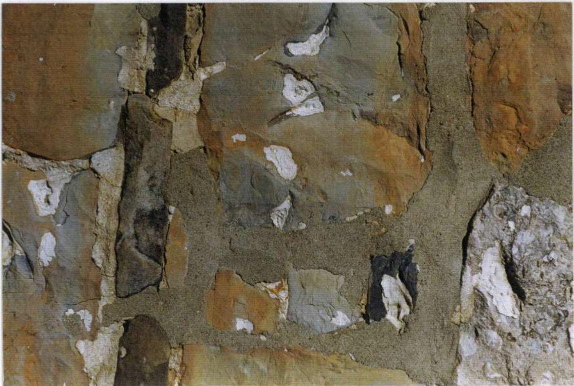
39. Phase three (phase five stone wall) with remains of whitewash finish.
