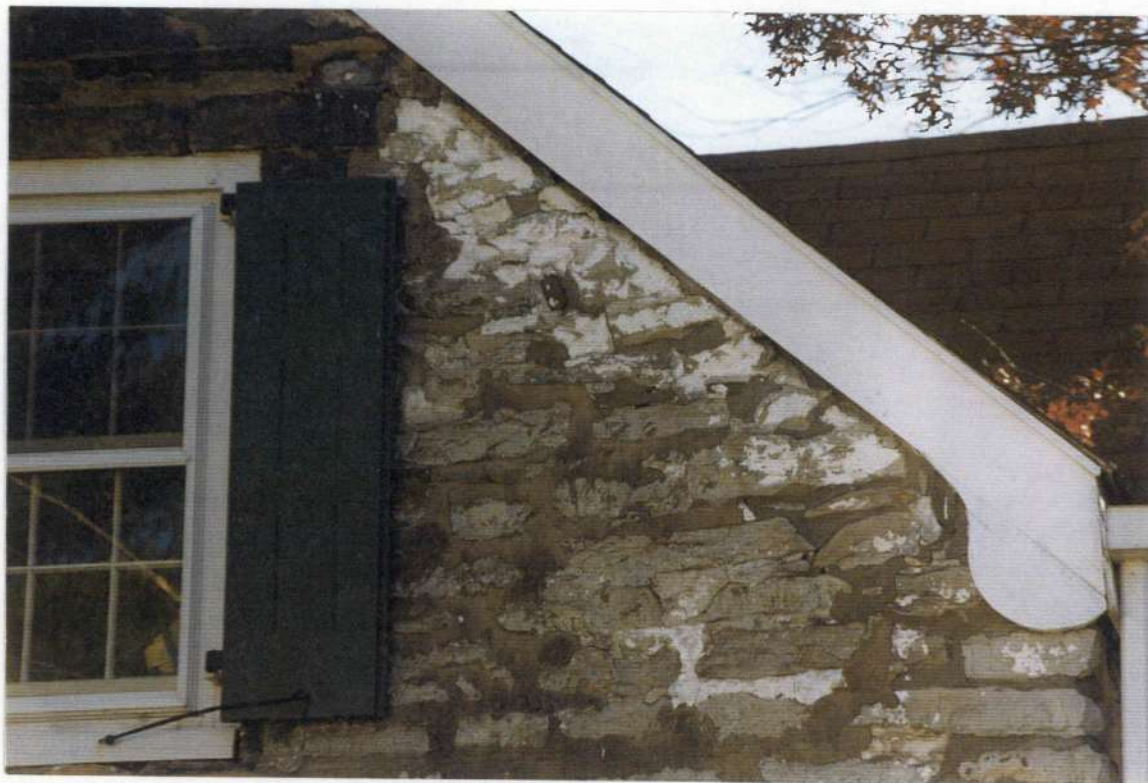
25. Detail: ca. 1970s cornice removed leaving pre-1850s whitewash.
