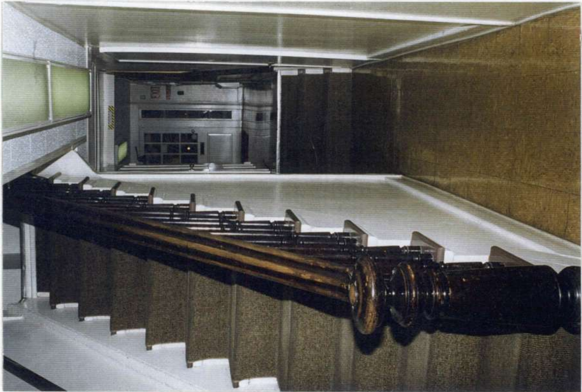
159. Space 107 stair hall. Stair and railing most likely not original.
