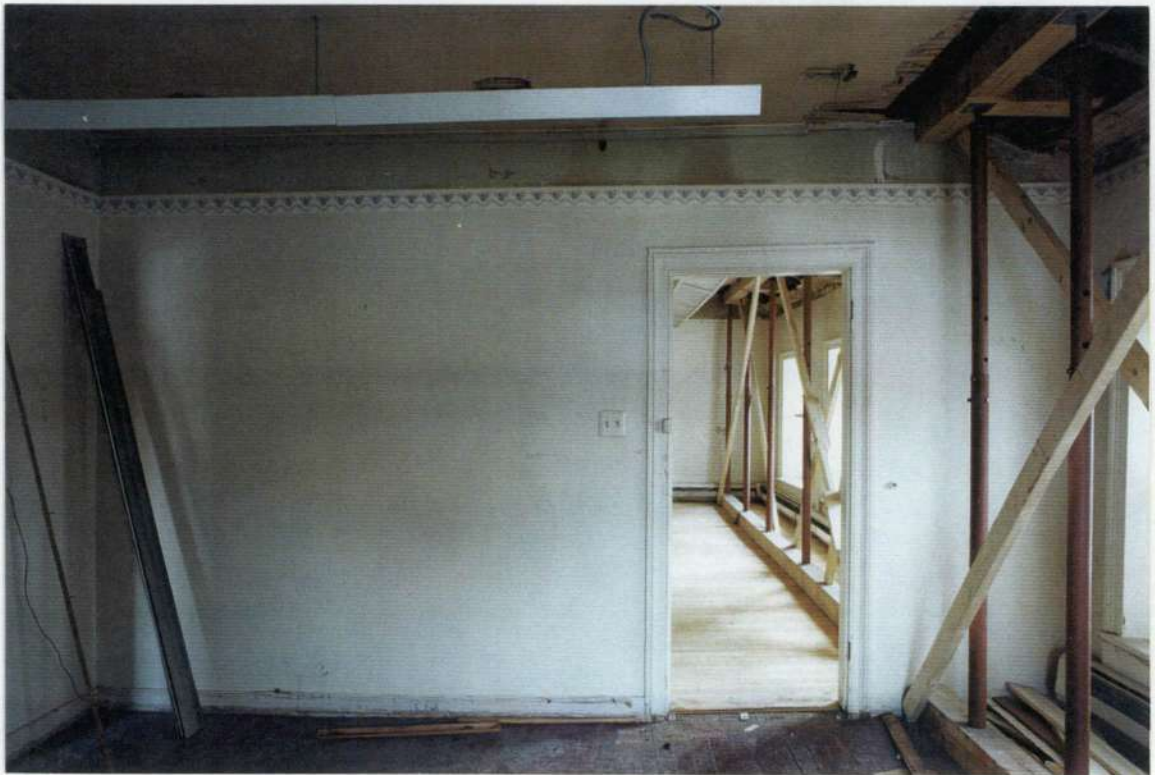
210. Space 207 west wall after removals.
