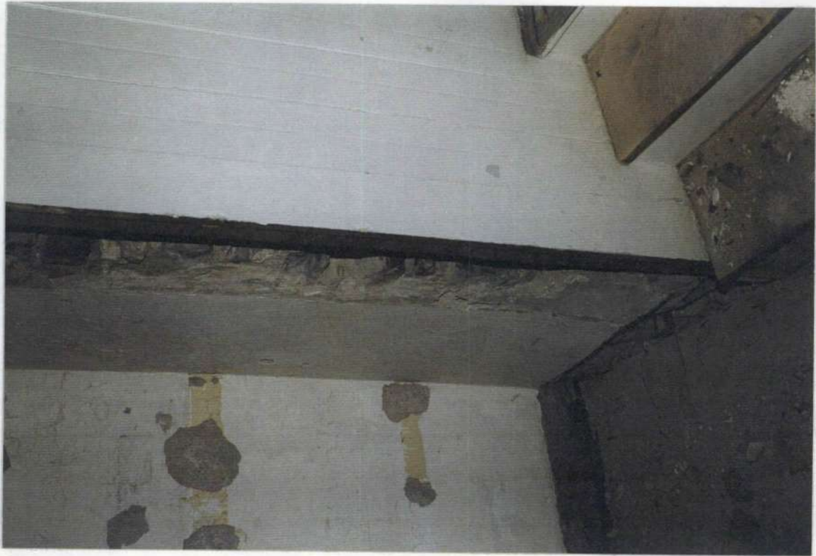
148i. Space 205 northeast corner of remains of phase four stone wall added to phase three east wall. Note ends of wide board plank flooring at stone wall.
