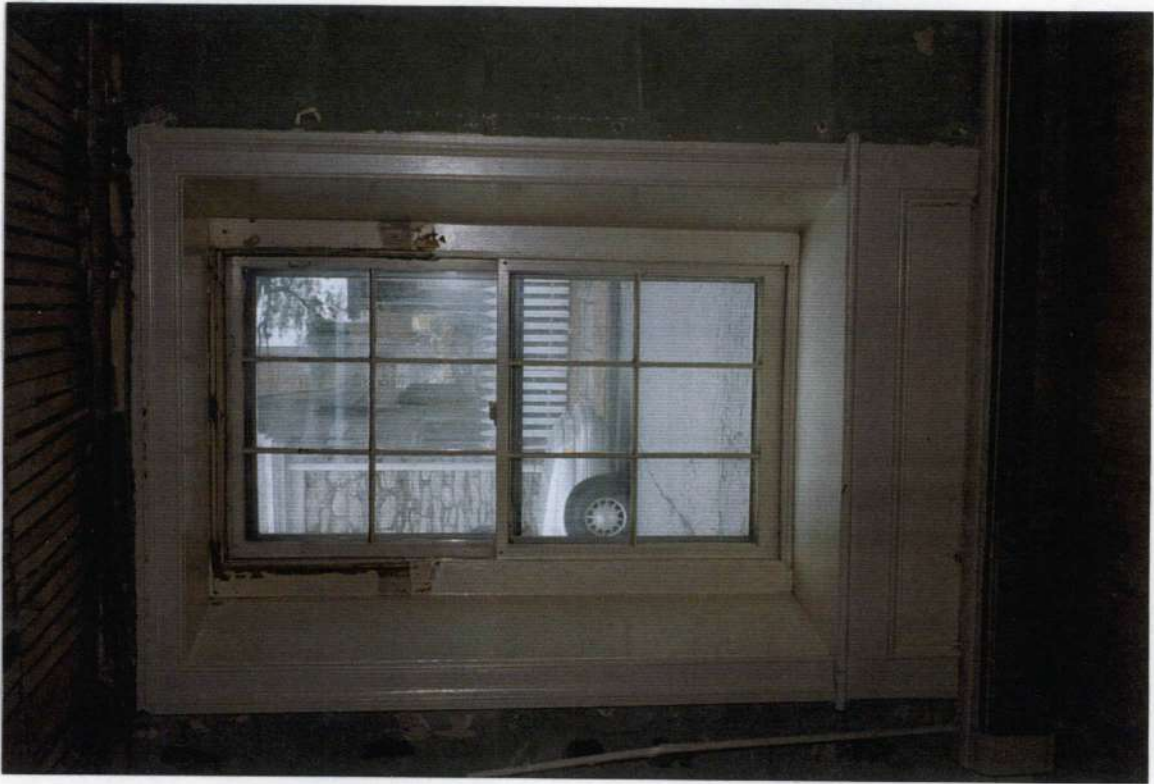
177. Space 108 north wall window.
