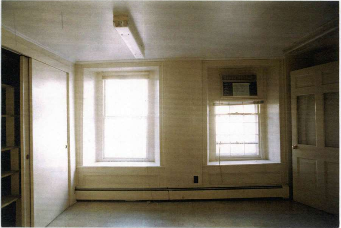
171. Space 105 north wall before removals.
