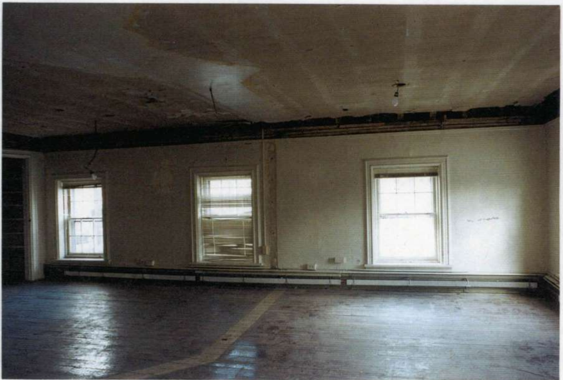
251. Space 215 and 216 north wall east wall after removals.
