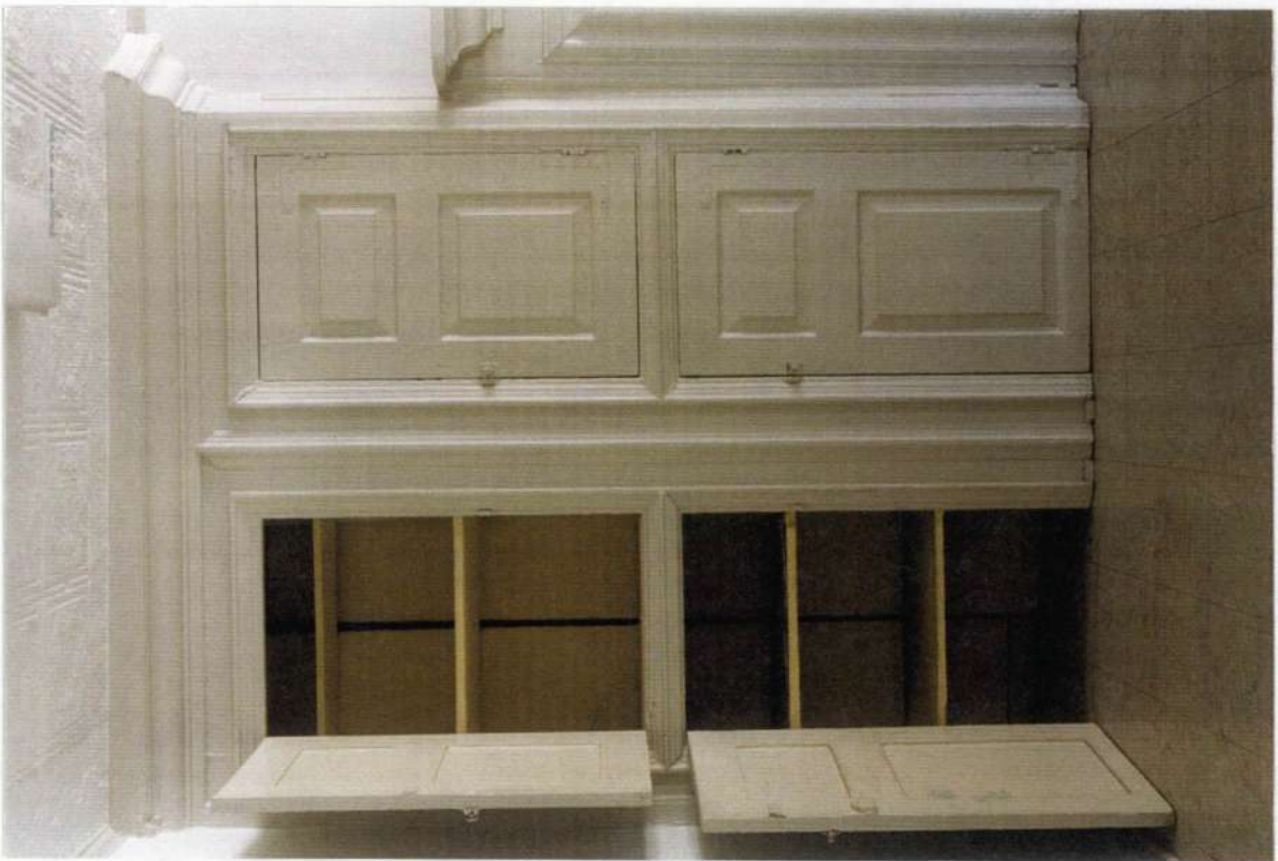
107. Detail: Cupboard opened position showing recessed flat panel detailing.
