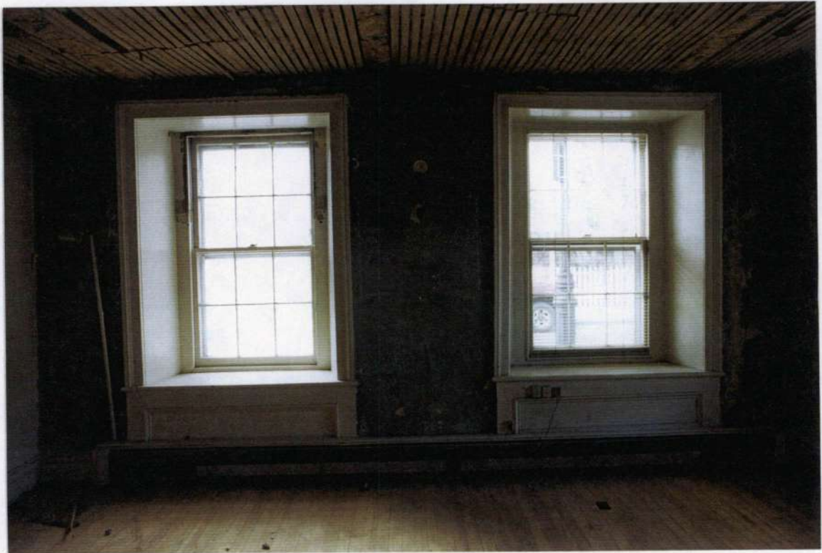
176. Space 108 north wall after removals.
