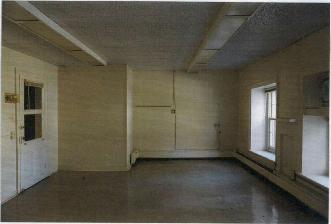
203. Space 206 west wall before removals.
