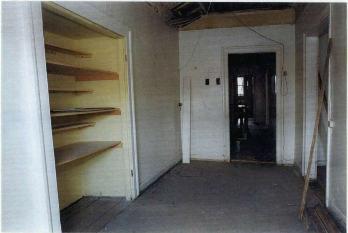
218. Space 208 south and west walls after removals.
