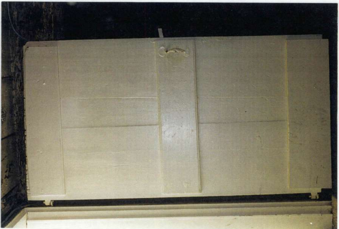
95. Space 104. Opposite side of door showing batten construction.
