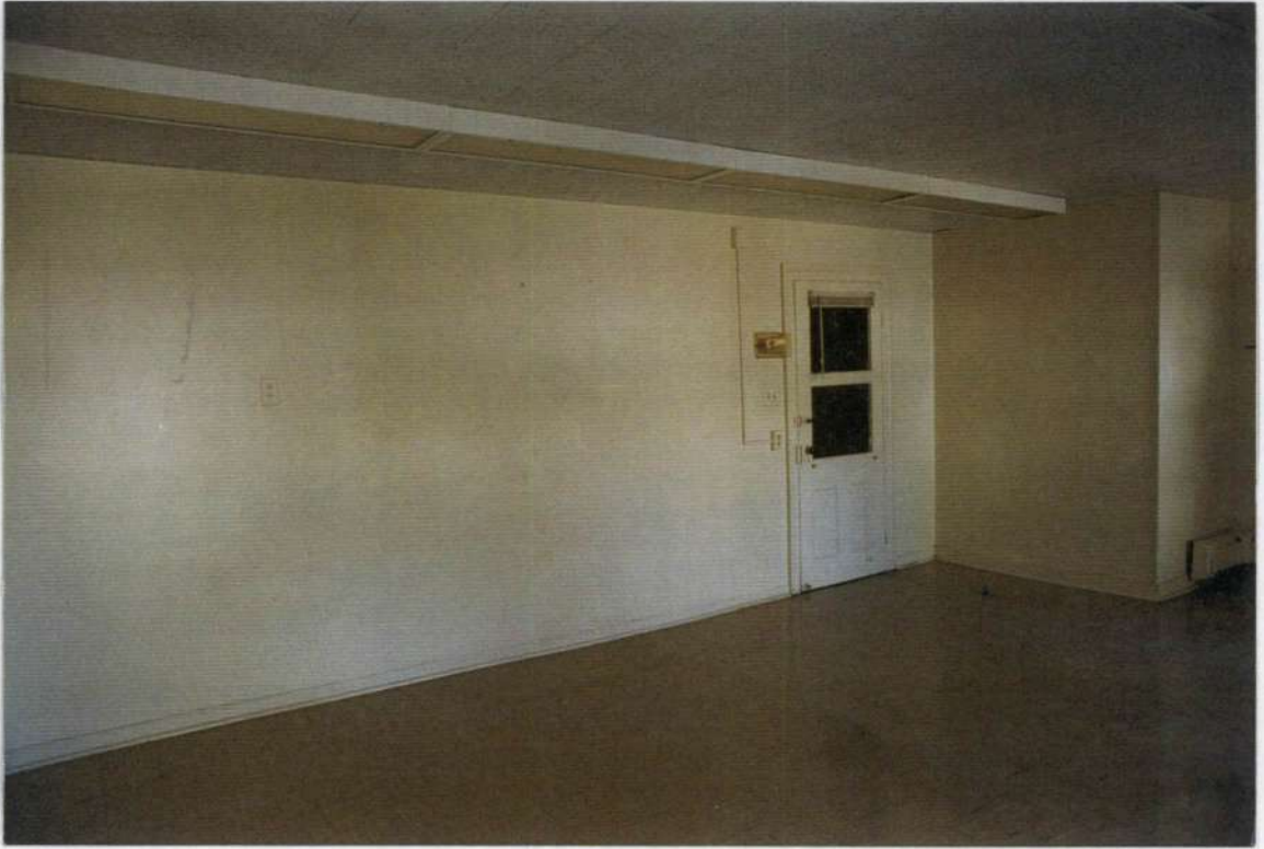
196. Space 206 south wall before removals.
