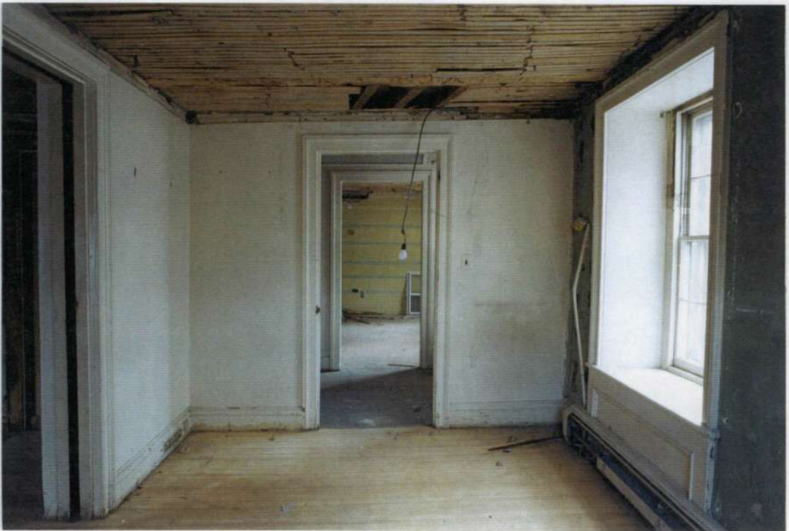
179. Space 108 west wall after removals.
