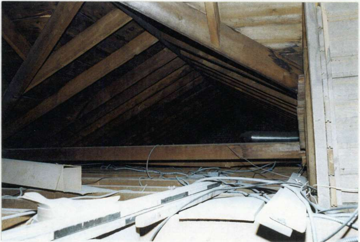
256. Attic from space 211 of phase five looking south.
