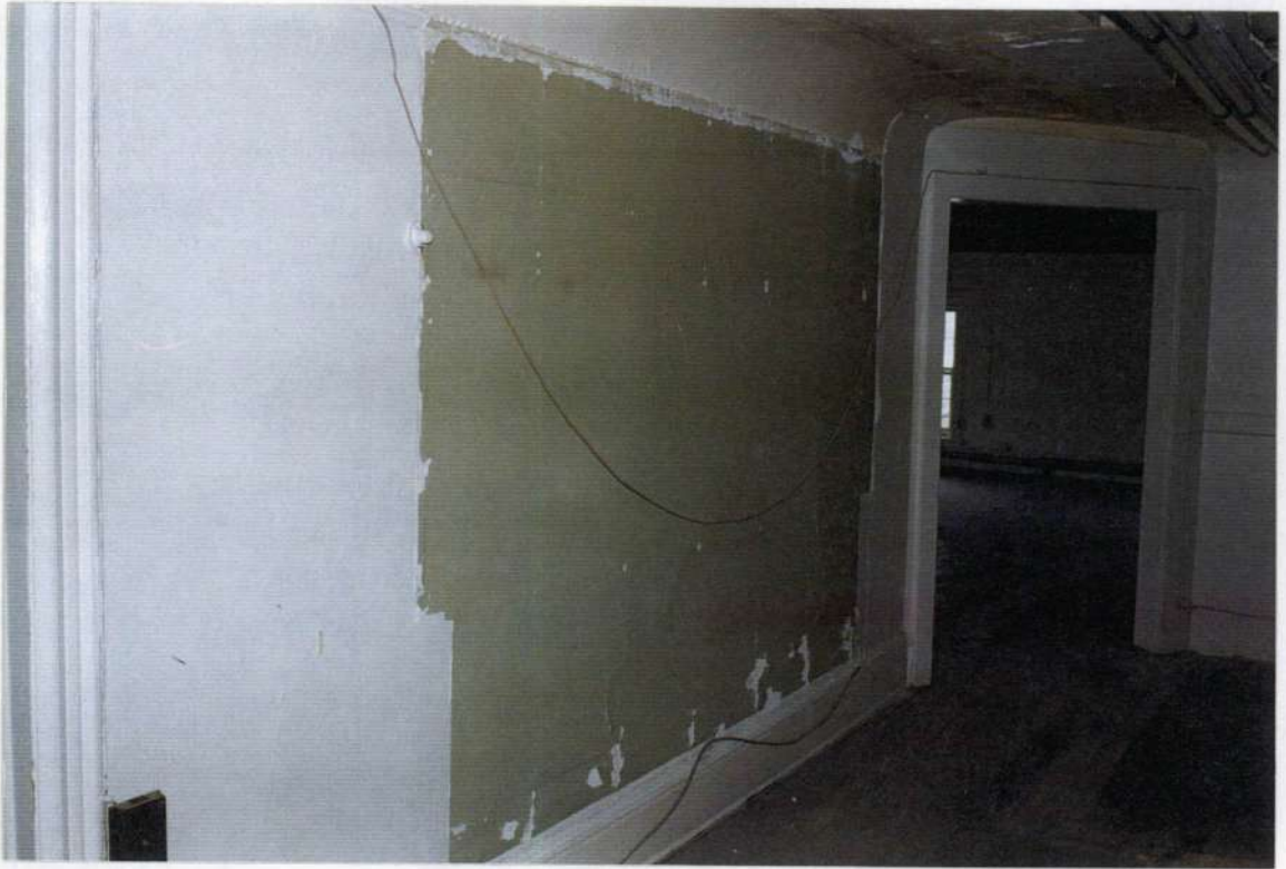
242. Space 211 east wall after removals. Note stairwell in floor.
