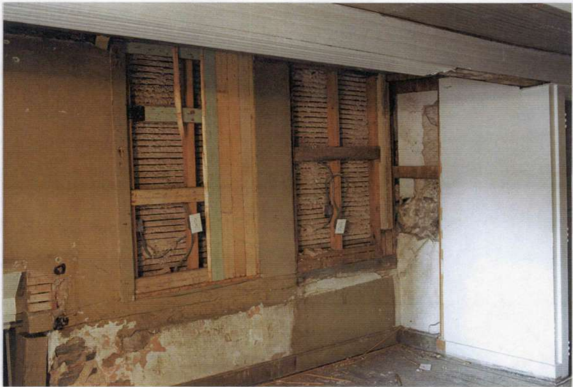
136. Detail: space 104 south wall, north end where stair up and down removed.
