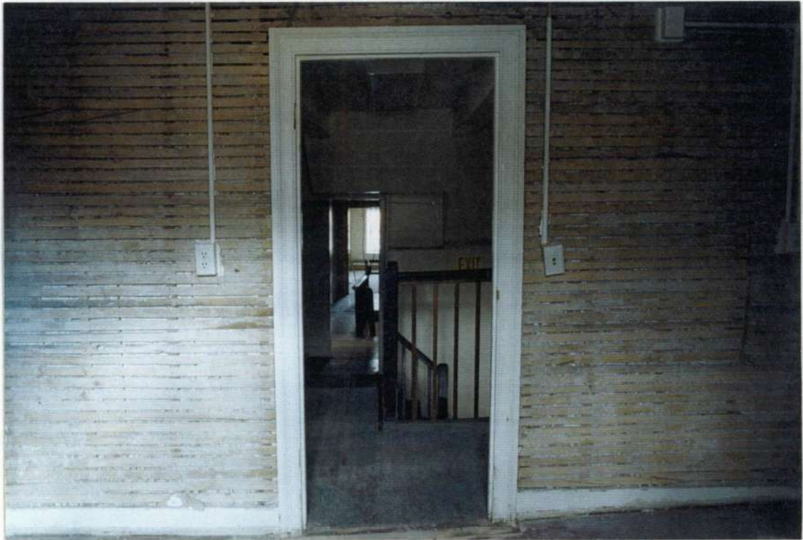
85. Space 203 east wall. Ca. 1850s wood lath and plaster applied over earlier vertical plank wall.
