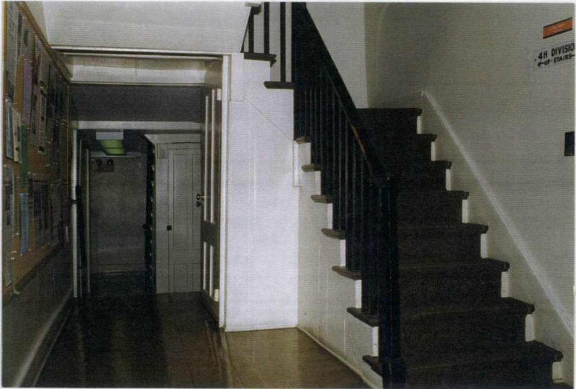
56. Space 102. Entry hall and stair looking east. Stone wall on right, vertical board wall below stair.
