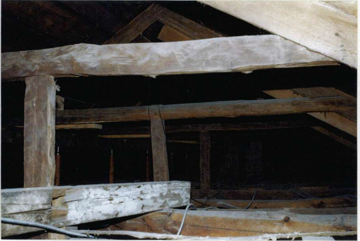
221. Attic over space 207 looking west.
