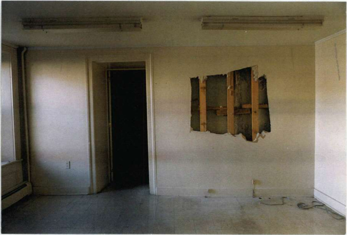
187. Space 109 south wall before removals.
