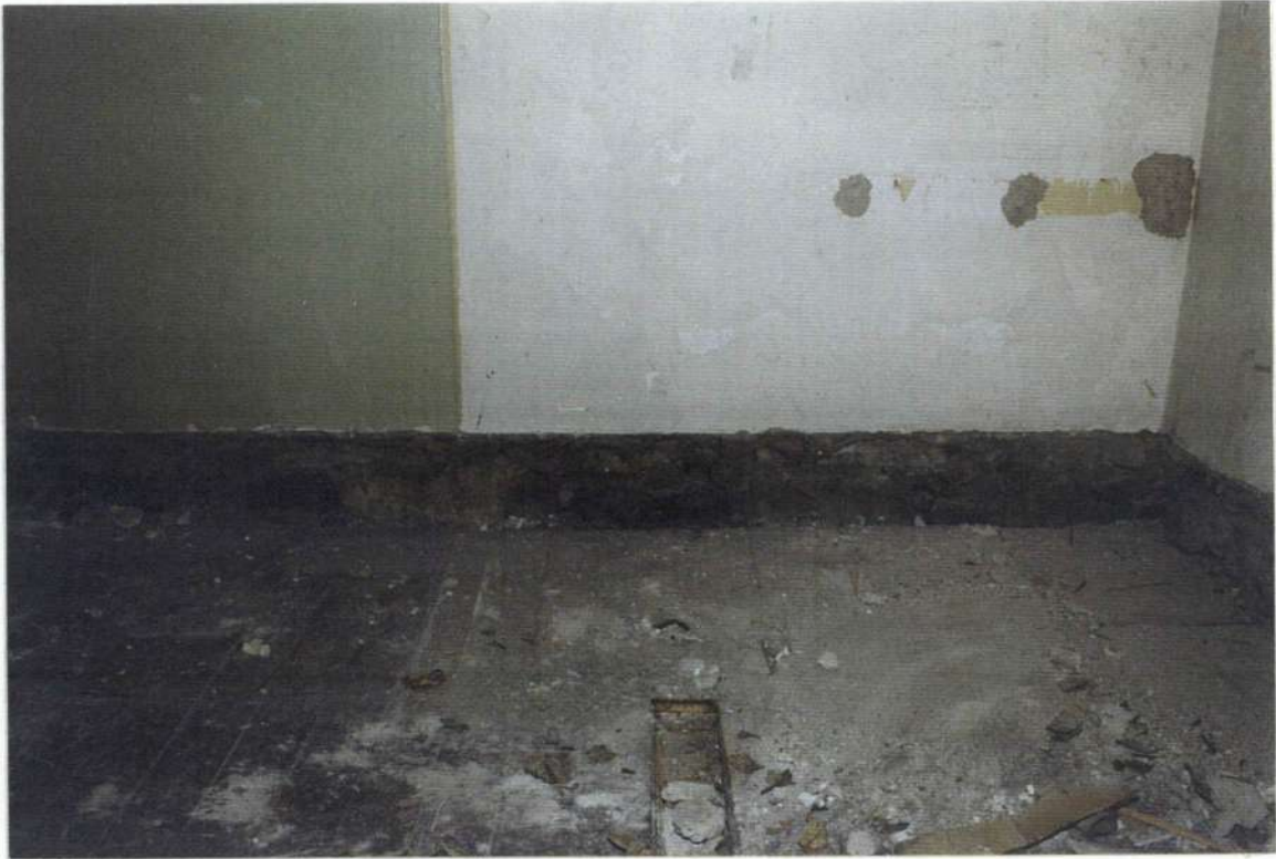
148g. Space 205 north wall. Baseboard removed. Burned stone, possible remains of burning in 1777.
