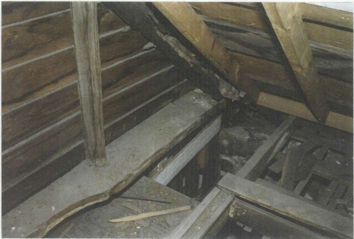
148t. Phase three attic over space 205, southeast corner. Note top of phase four stone wall, and phase four gable end wall plate with wood clapboard on outside. Note earlier phase three end hand-hewn rafter at clapboard.
