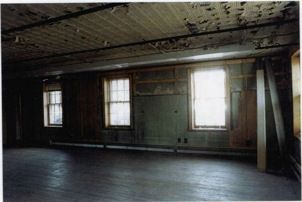
237. Space 113 east wall after removals.
