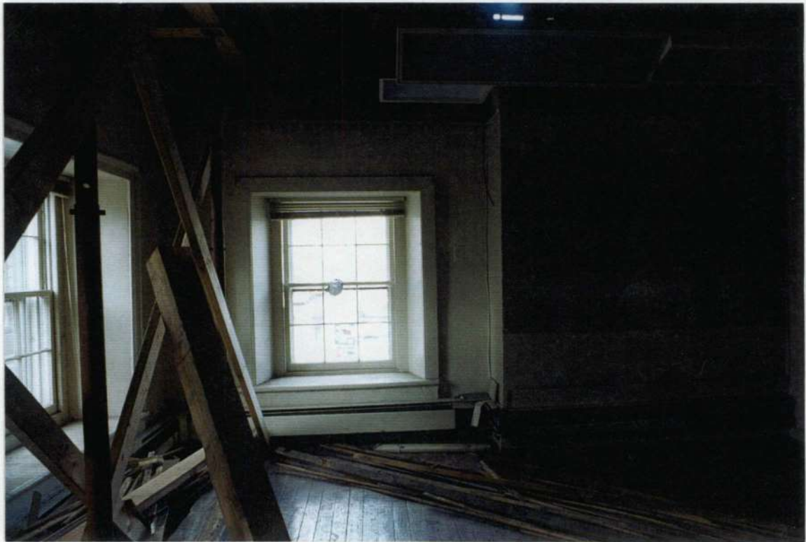
206. Space 207 east wall after removals.
