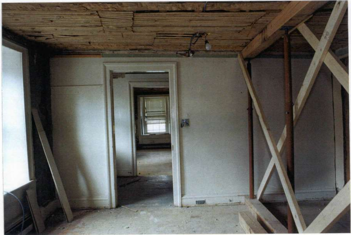
169. Space 105 east wall after removals.
