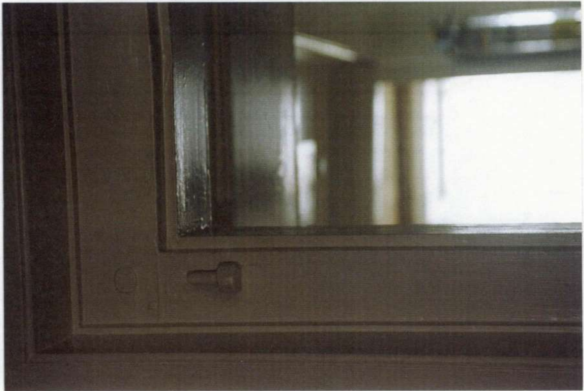
67. Detail of mortise and tenon pegged detail door frame with pintel in stone wall between phases one and four.
