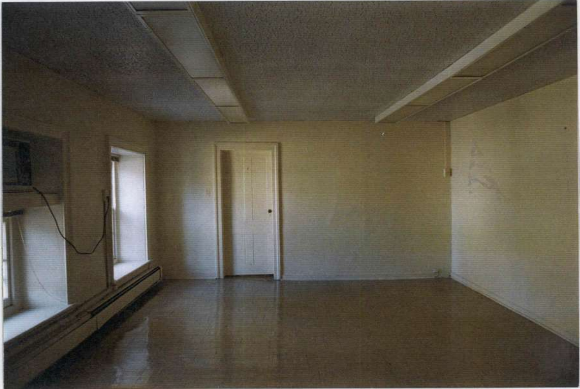
199. Space 206 east wall before removals.
