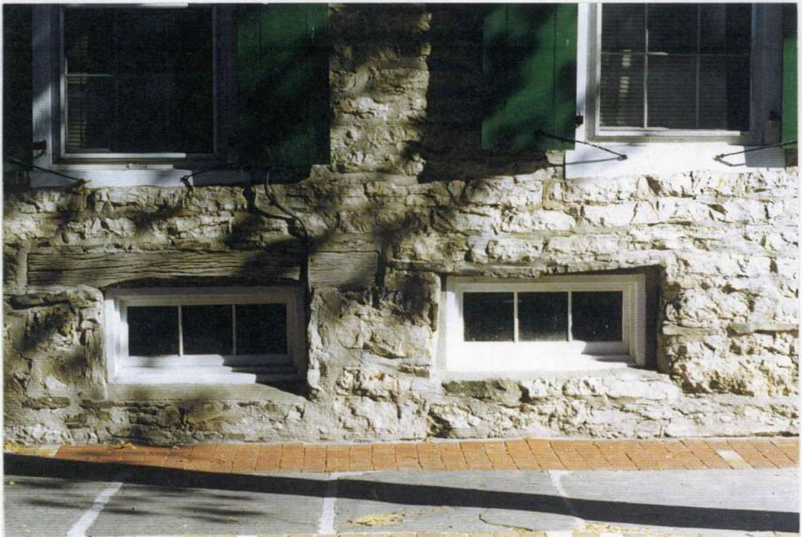
19. Cellar window to south of entry door. Note timber lintel over left window, earlier door to exterior.
