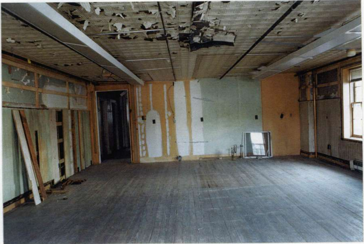
236. Space 113 north wall after removals.
