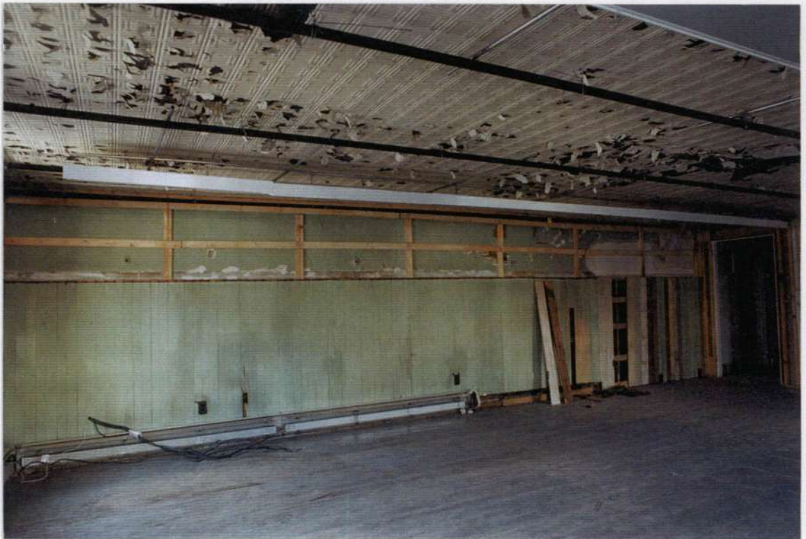
235. Space 113 west wall after removals.
