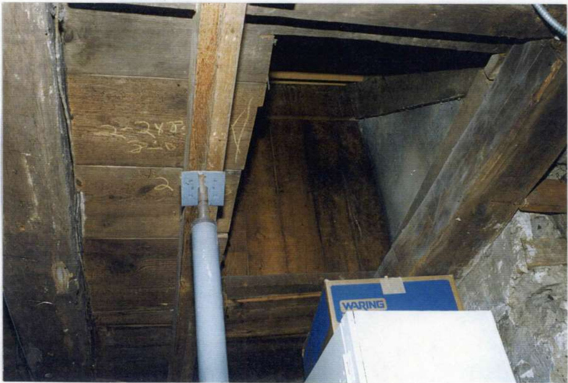
43. Space 001 southeast corner. Earlier stair opening to first floor (below present stair).
