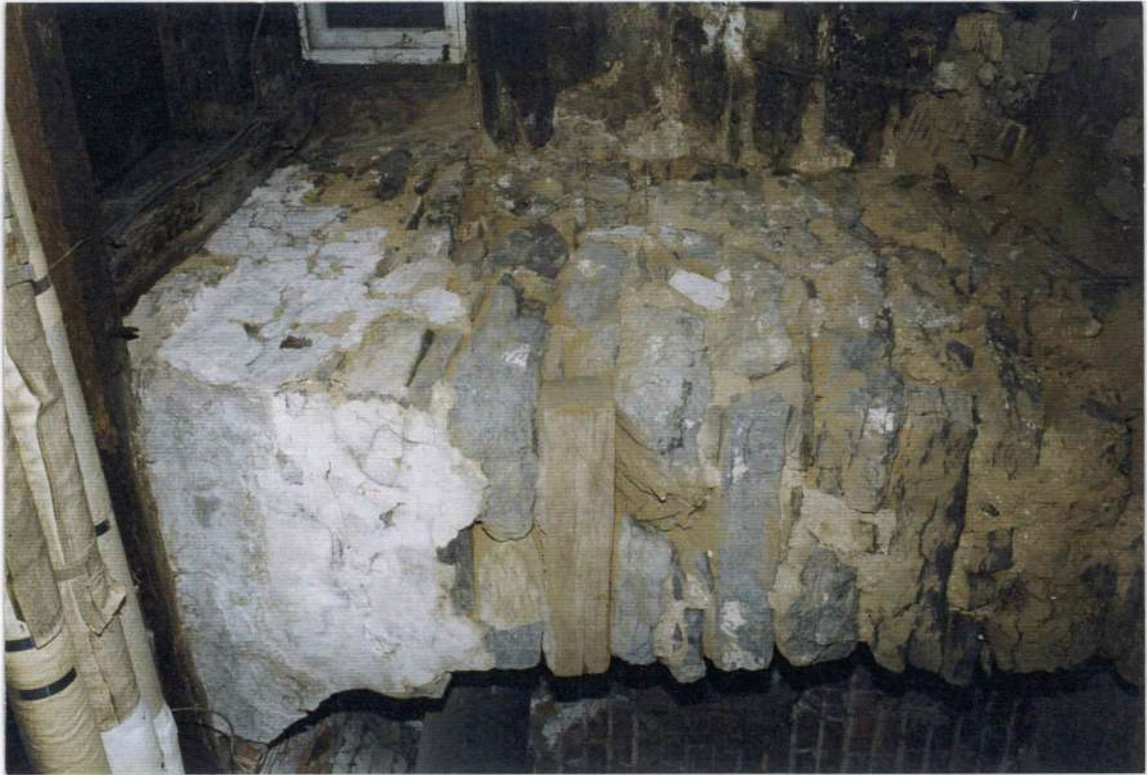
158. Space 003 east wall fireplace foundation.
