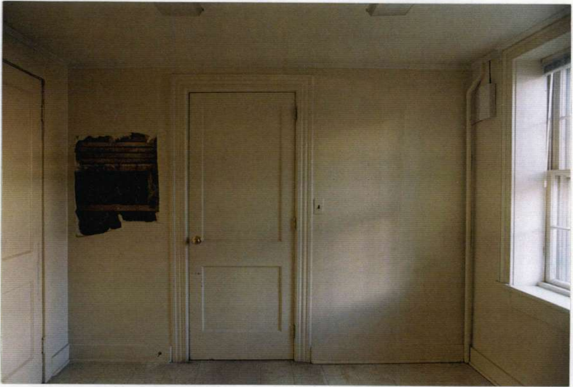
225. Space 112 north wall before removals.
