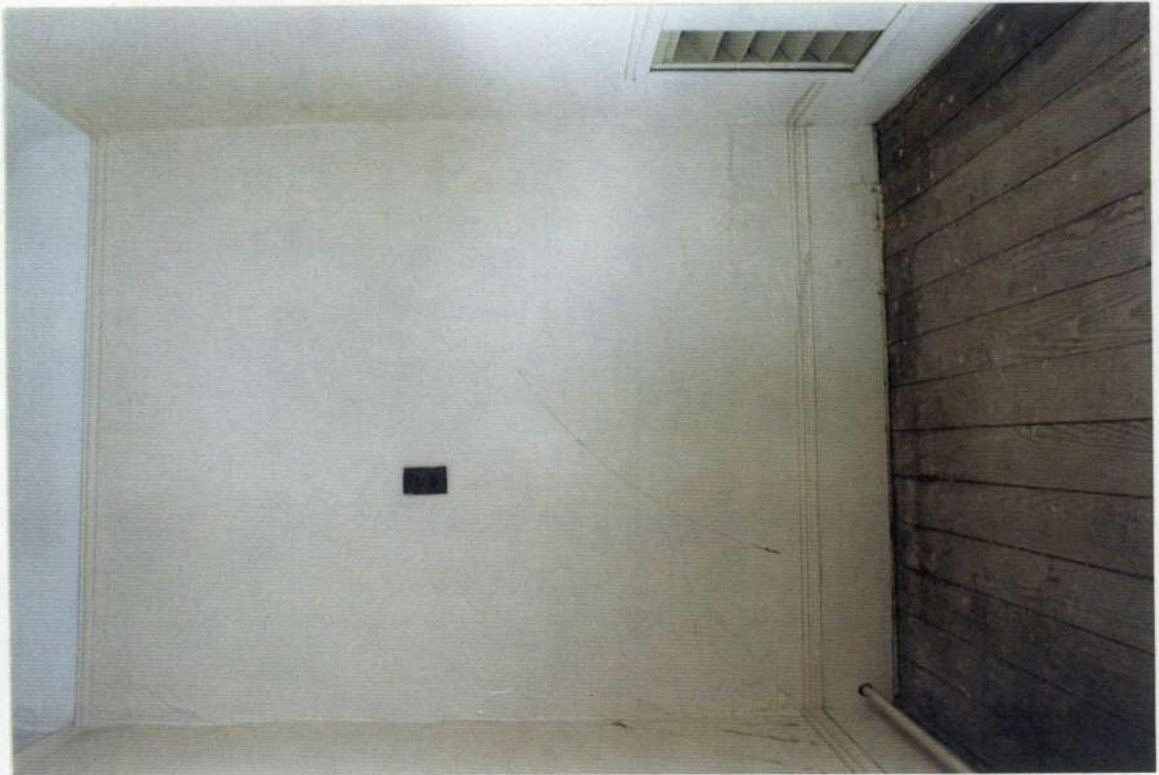
253. Space 214 north wall after removals.
