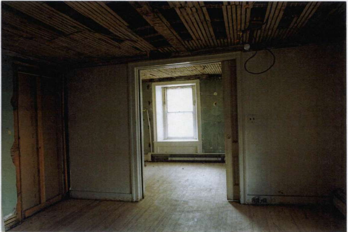
184. Space 109 north wall after removals.
