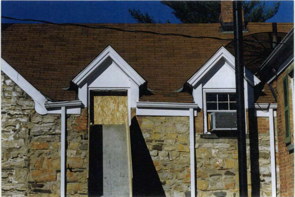
32. Stone infill wall phase three (phase five stone wall). Gable-ended dormers added phase five. This non-limestone wall was whitewashed to match earlier finish of stonework.
