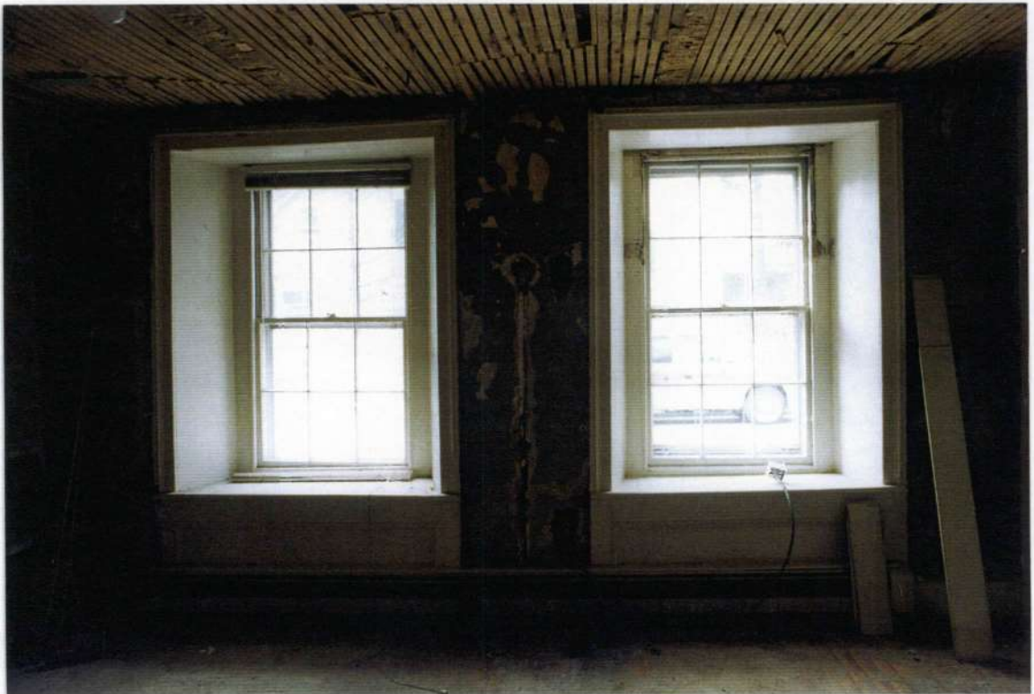
172. Space 105 north wall after removals.
