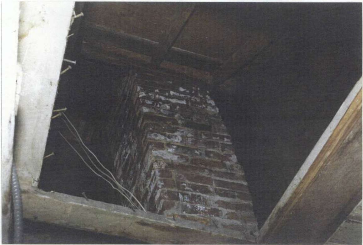
148o. Space 205. Top of early chimney in east wall attic.
