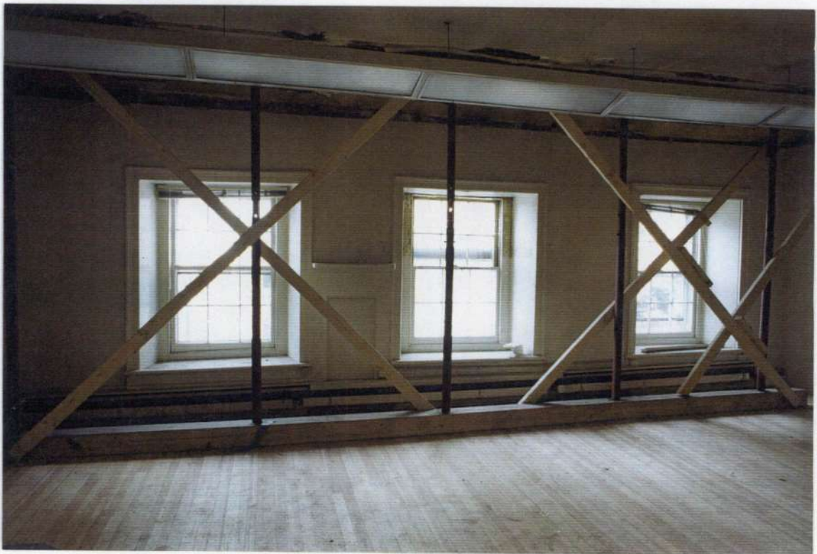
202. Space 206 north wall after removals.
