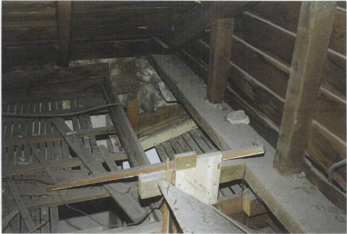
148s. Phase three attic over space 205, northeast corner. Note top of phase four stone wall and phase four gable end wall plate with wood clapboards on the outside.
