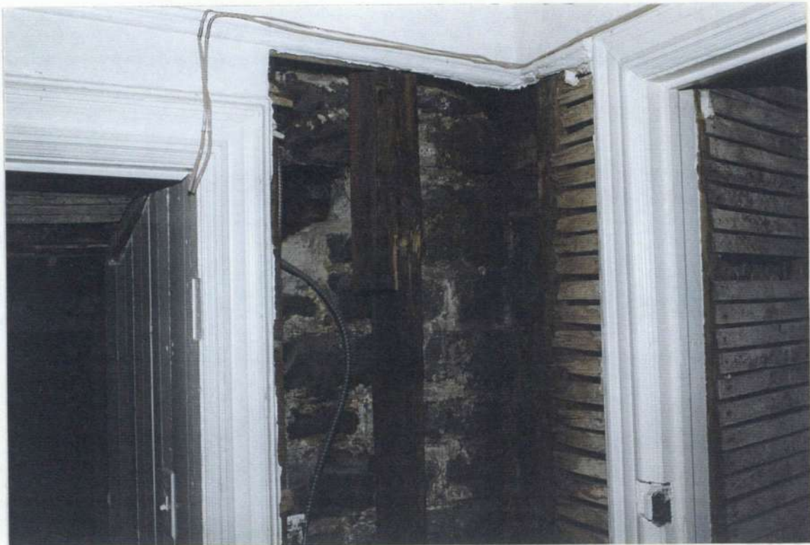
153b. Northeast corner of phase four stone wall added to east wall of phase three. As seen from phase five. This is the junction at the phase four south wall.
