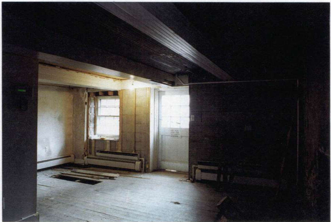
133. Space 104 south wall after removals.
