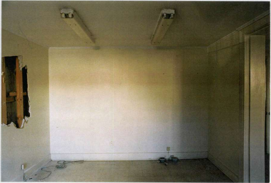
185. Space 109 west wall before removals.
