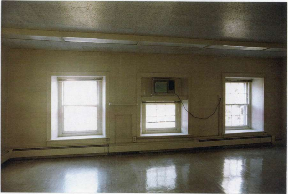
201. Space 206 north wall before removals.
