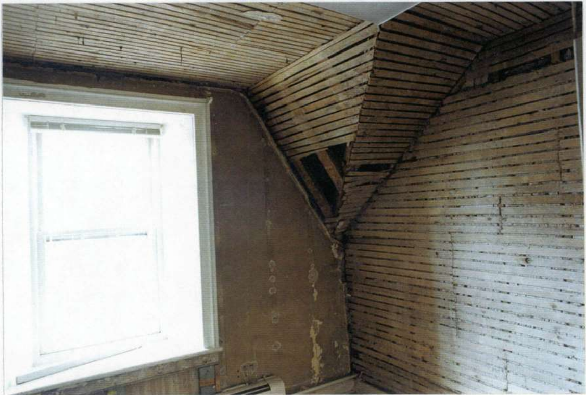
88. Space 203 west wall. Note plastered exterior stone wall; higher window of ca. 1850s ceiling in this space was raised above the wood plank ceiling of other phase one spaces. This space would not have had a window before this period.
