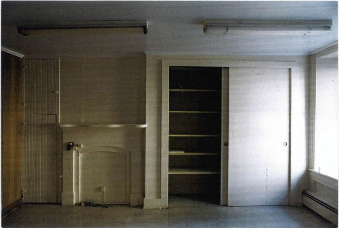
162. Space 105 west wall before removals.
