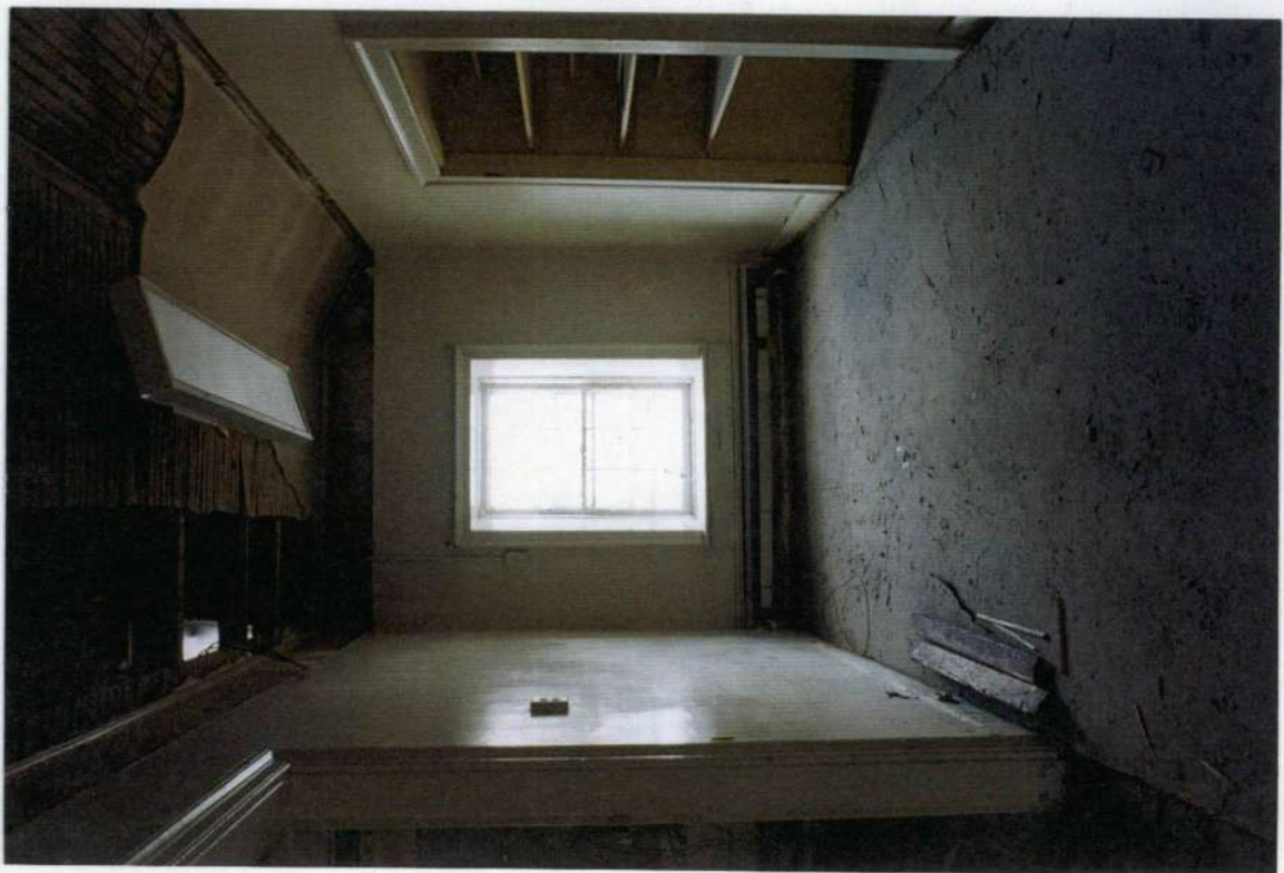
216. Space 208 east wall after removals.
