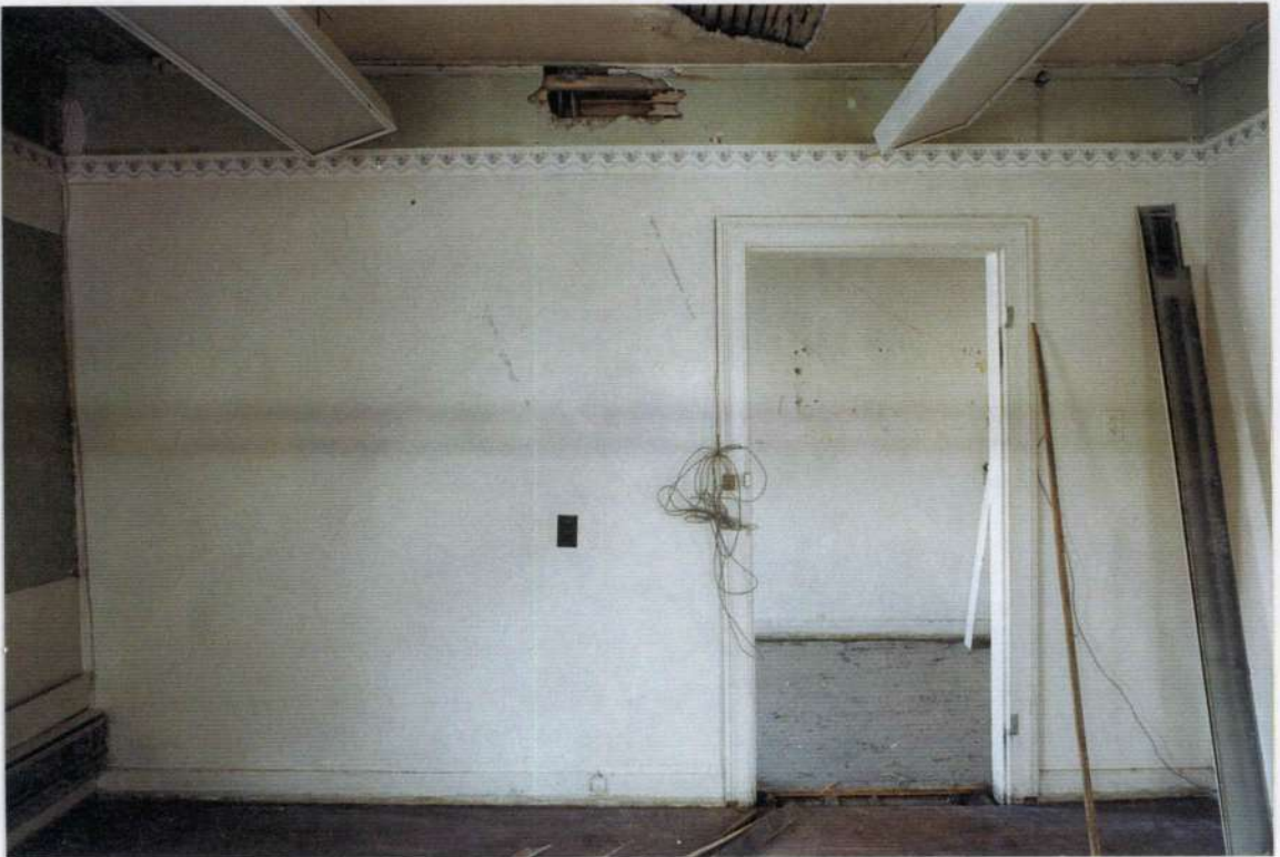
212. Space 207 south wall after removals.
