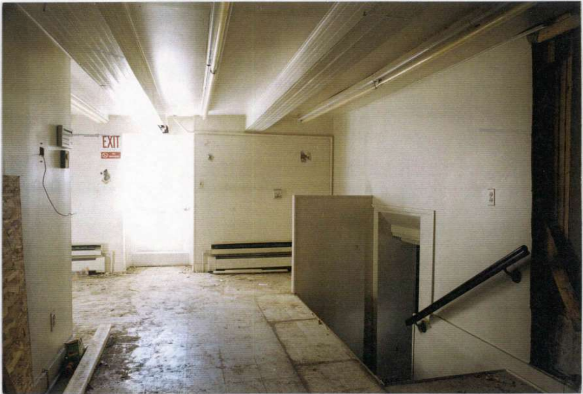
130. Space 104 south wall before removals.
