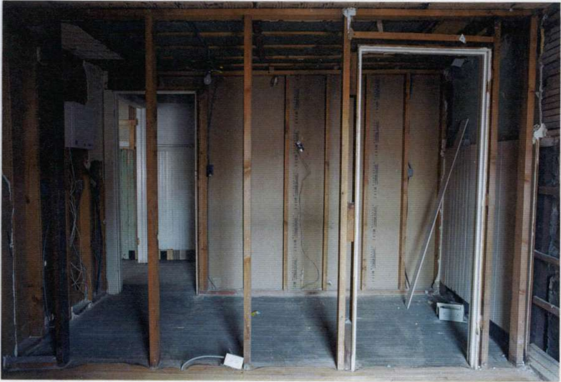
227. Space 112 west wall after removals.
