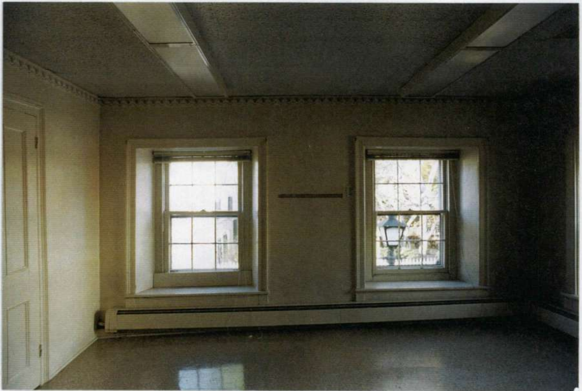
207. Space 207 north wall before removals.
