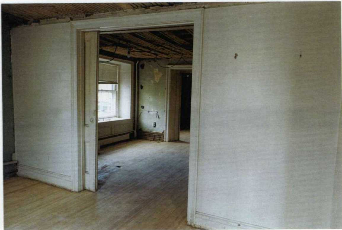
181. Space 108 south wall after removals.
