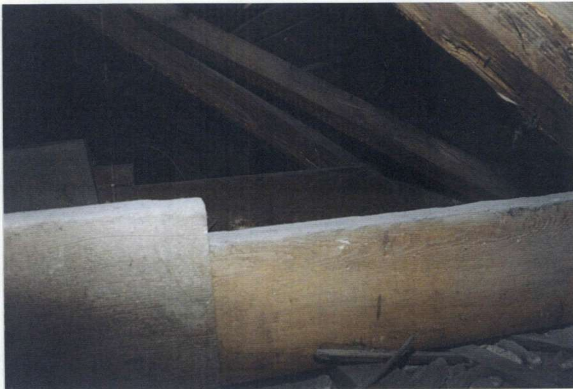
150a. Space 205 attic from southeast corner looking east. Note spliced ceiling rafters to hand-hewn early roof rafters.
