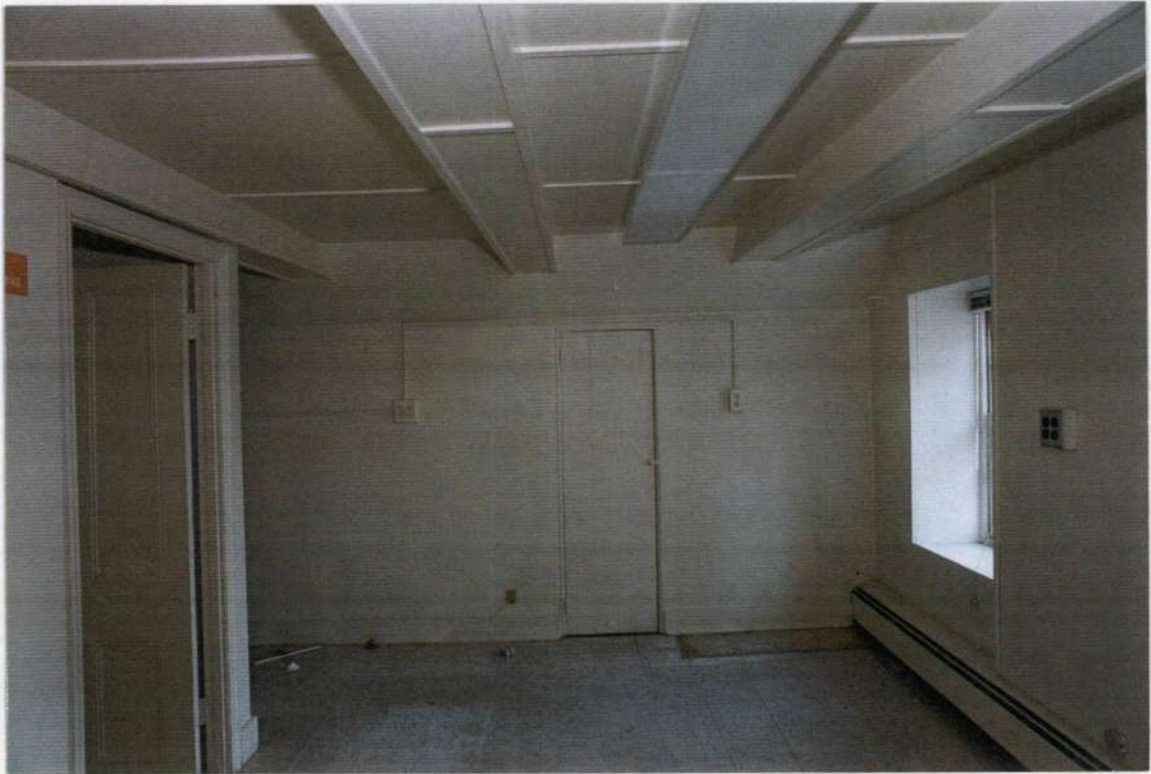
75. Space 201. West wall before removals.
