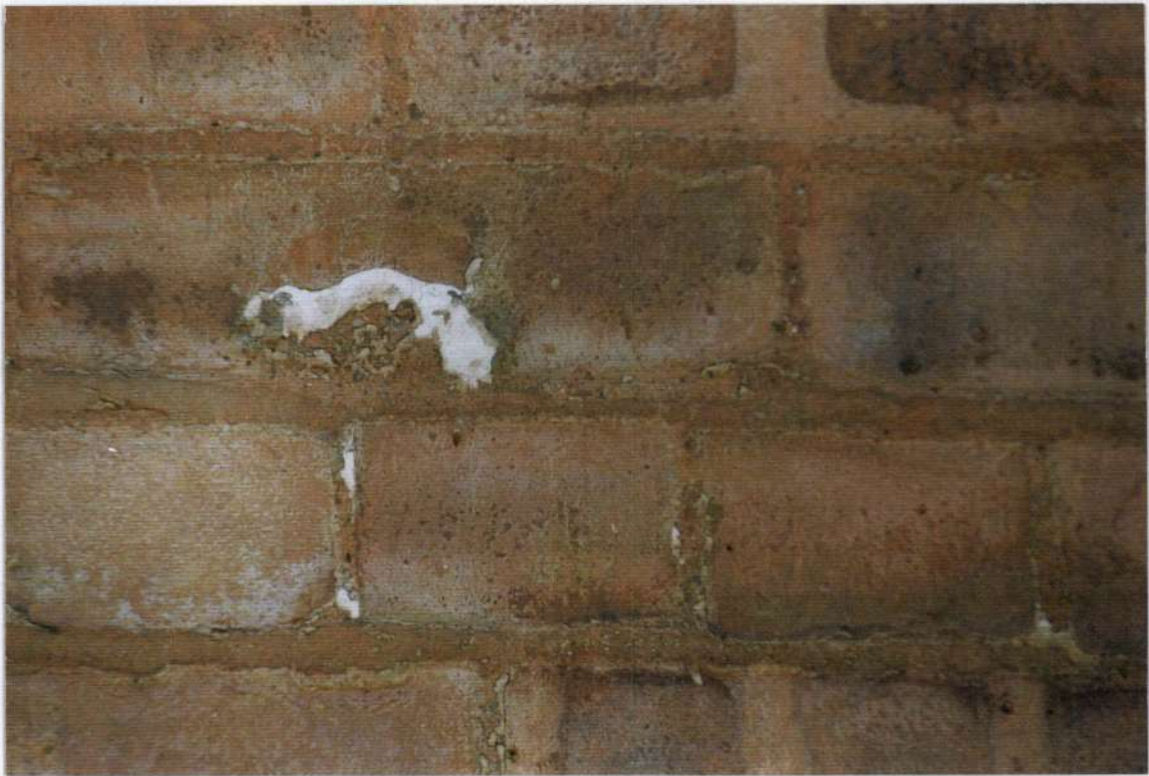
38. Phase five brick addition indicating painted or whitewashed wall.
