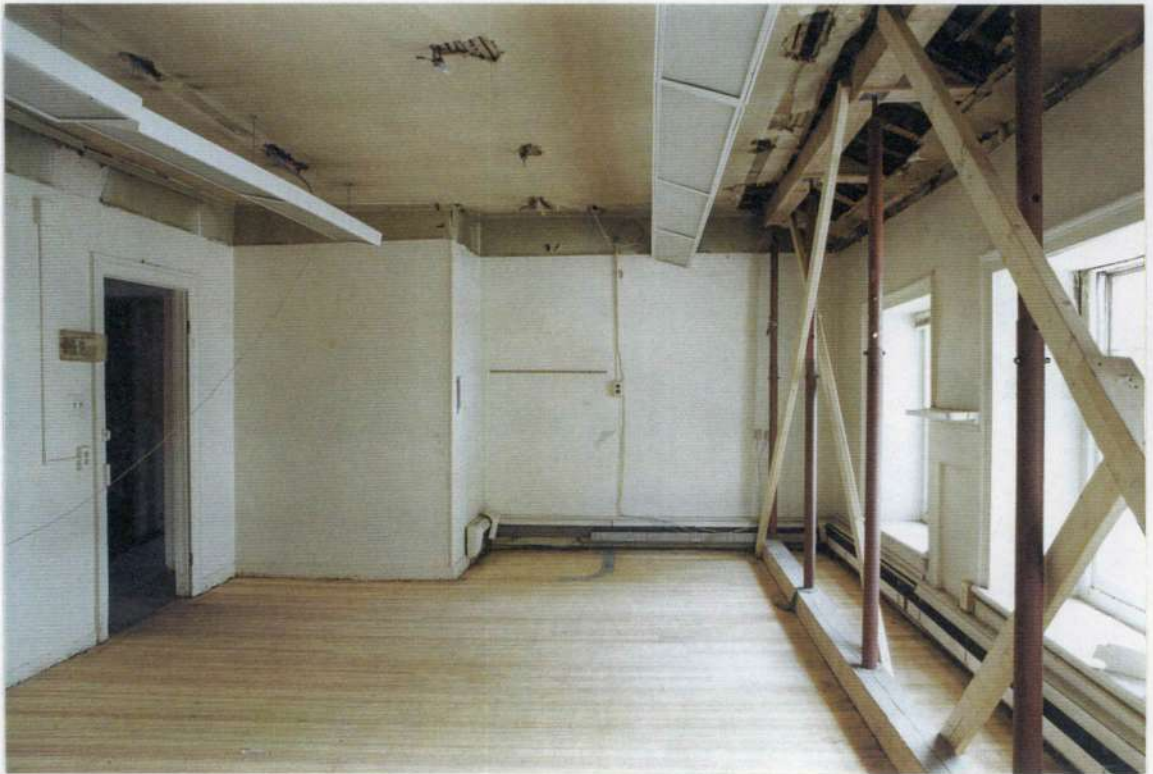
204. Space 206 west wall after removals.
