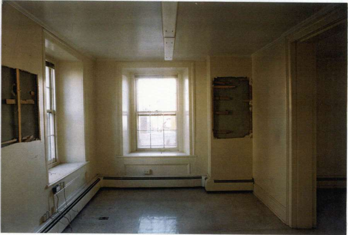
173. Space 108 east wall before removals.
