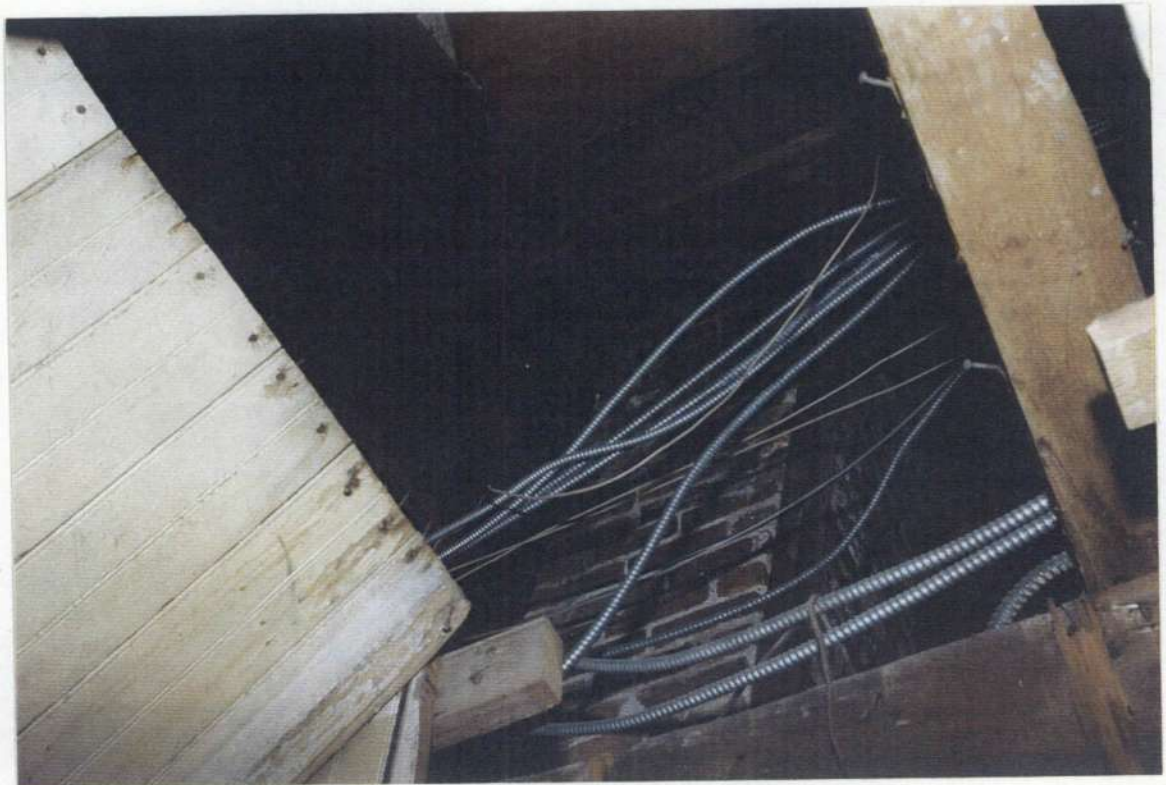
148p. Space 205. Top of early chimney in east wall attic.
