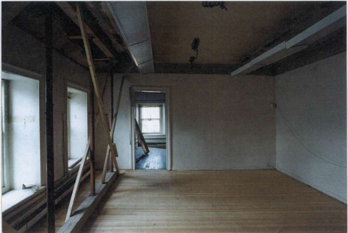
200. Space 206 east wall after removals. Note emergency roof shoring.
