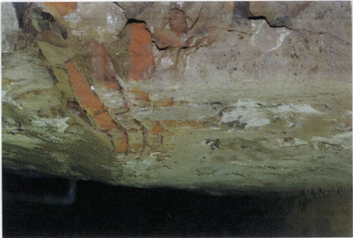
41. Detail of remains of arched brick.
