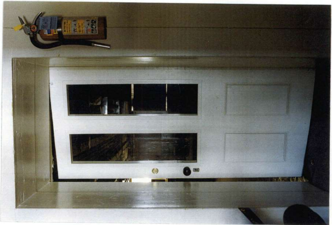
141. Door to space 205 from space 210.
