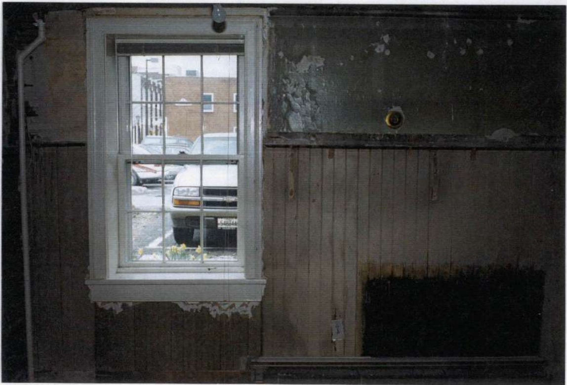
231. Space 112 east wall after removals.
