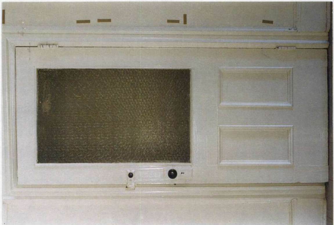
247. Door to closet in north wall of space 211.
