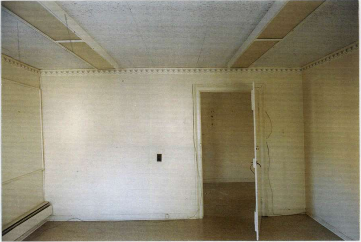
211. Space 207 south wall before removals.
