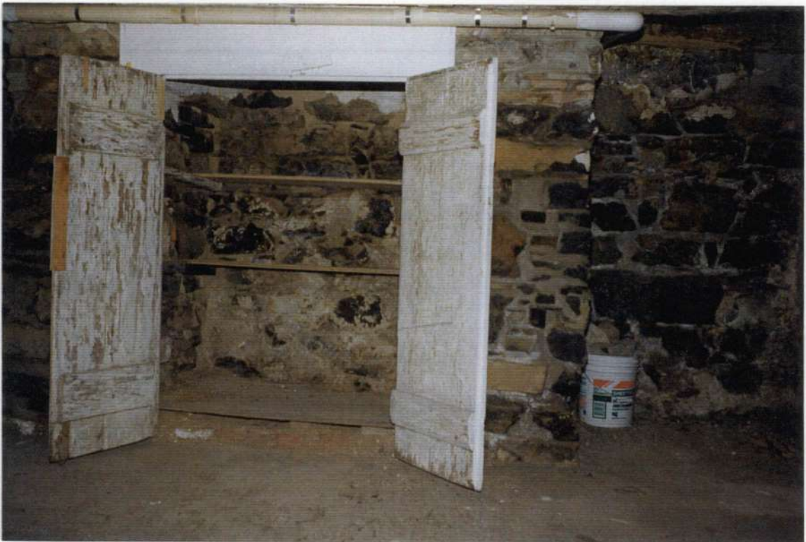
103. Interior of fireplace foundation.
