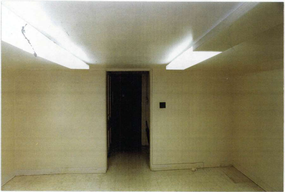
118. Space 204. North wall before removals.
