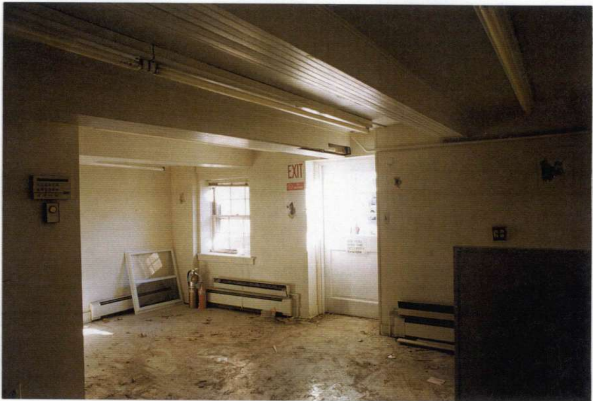
132. Space 104 south wall before removals.
