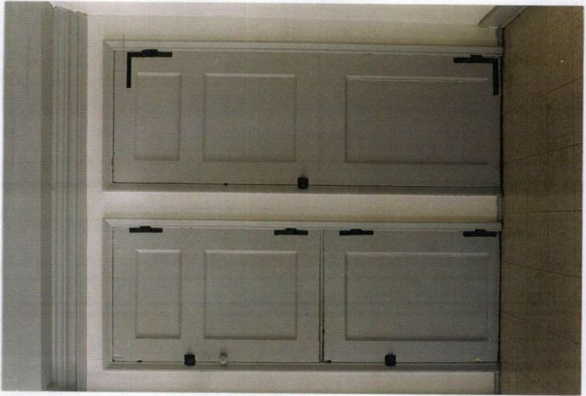
48. Fireplace cupboards. Flat panel detailing.
