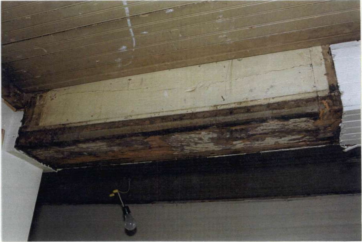
138. Detail: original beam showing the stair construction attachment and painted first riser down from the second floor of phase three to the first floor of phase two.
