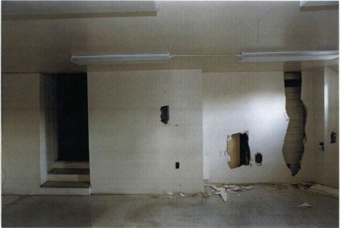
147. Space 205 east wall before removals.
