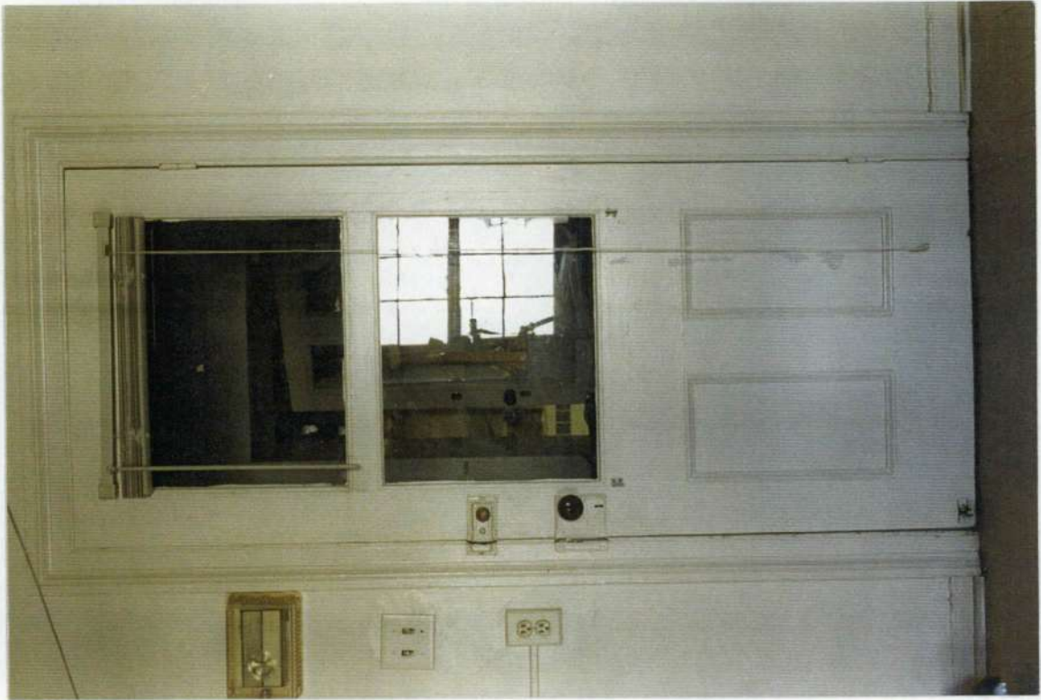
198. Door between space 206 and 210.
