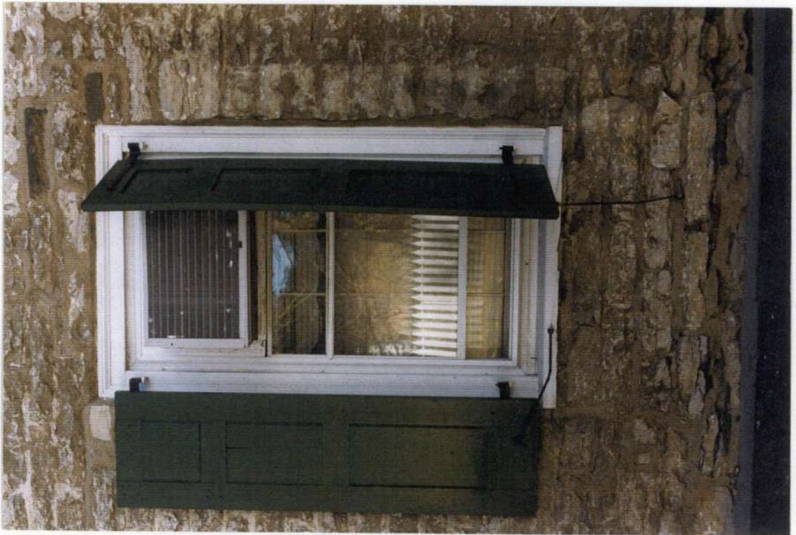
29. Typical replacement window and shutters and aluminum storm windows.
