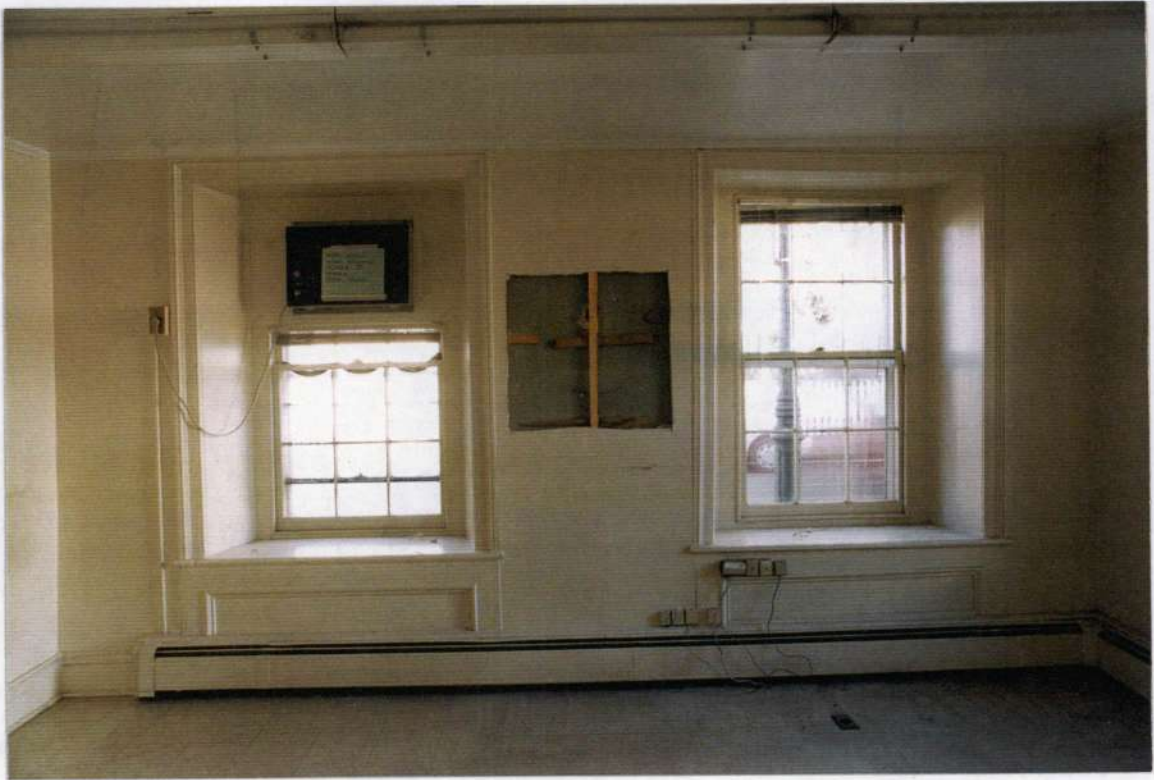
175. Space 108 north wall before removals.
