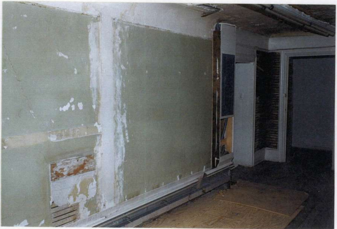
243. Space 211 west wall after removals.
