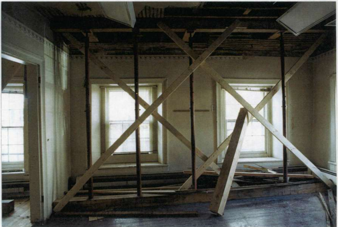
208. Space 207 north wall after removals.
