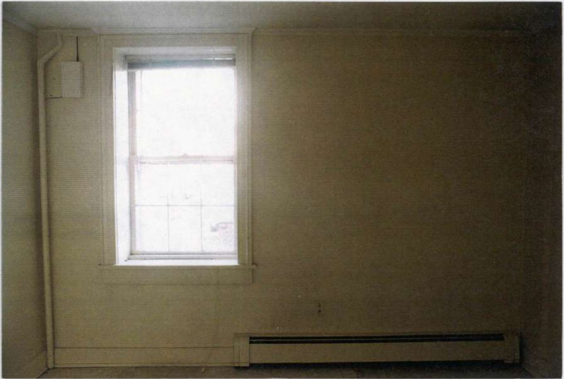
230. Space 112 east wall before removals.
