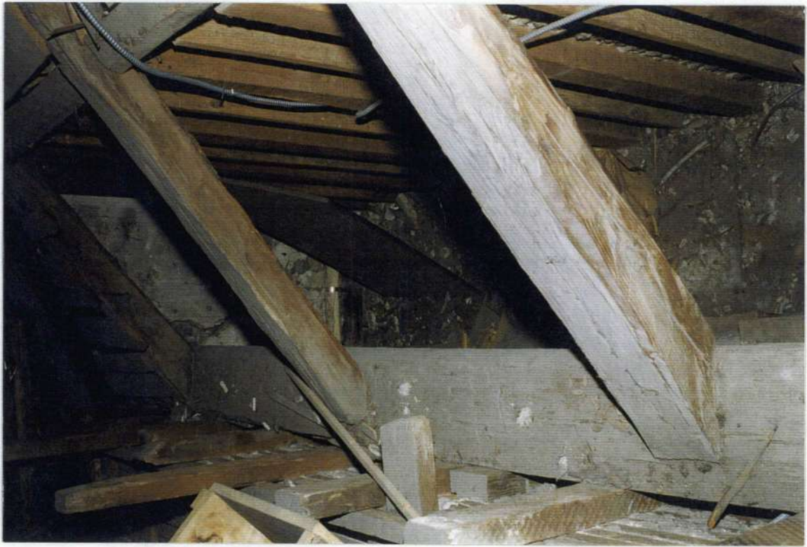
129. Space 204B view from above rafters and timber sill looking south.
