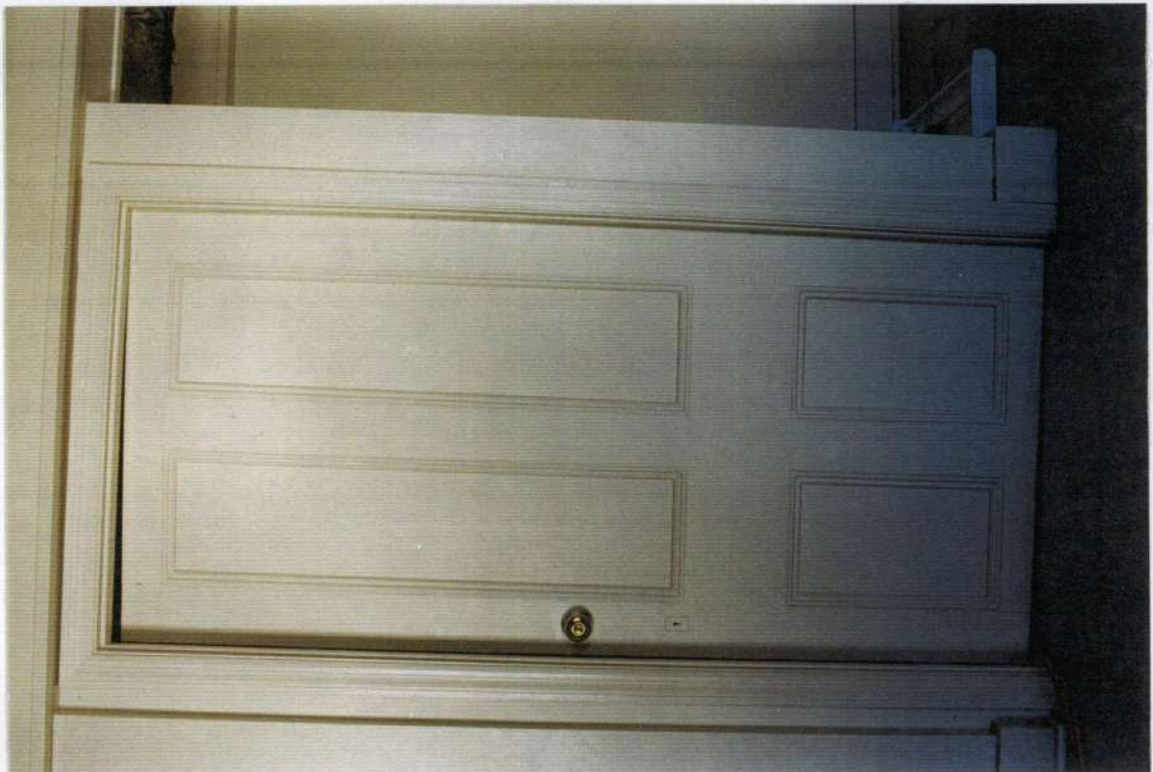
68a. Door between space 201 and 201a.
