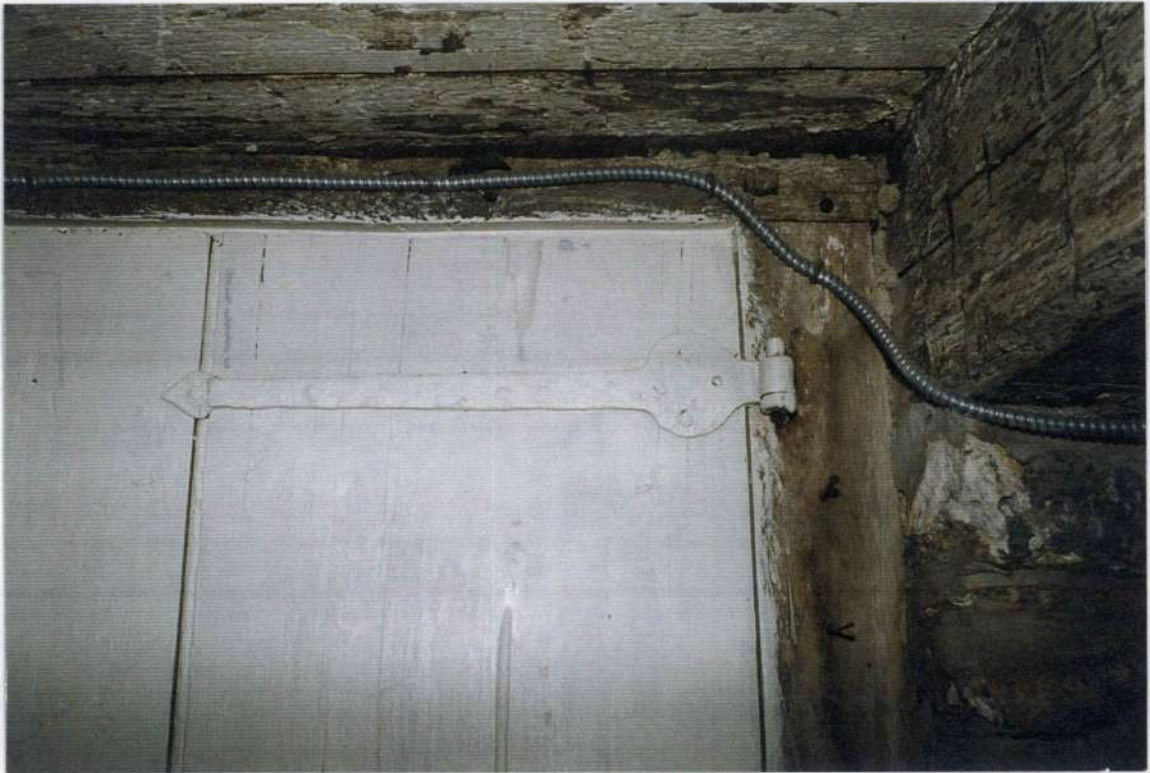
96. Detail: Wrought iron Dutch pancake strap and pintel hinge with mortise and tenon pegged heavy timber door frame.
