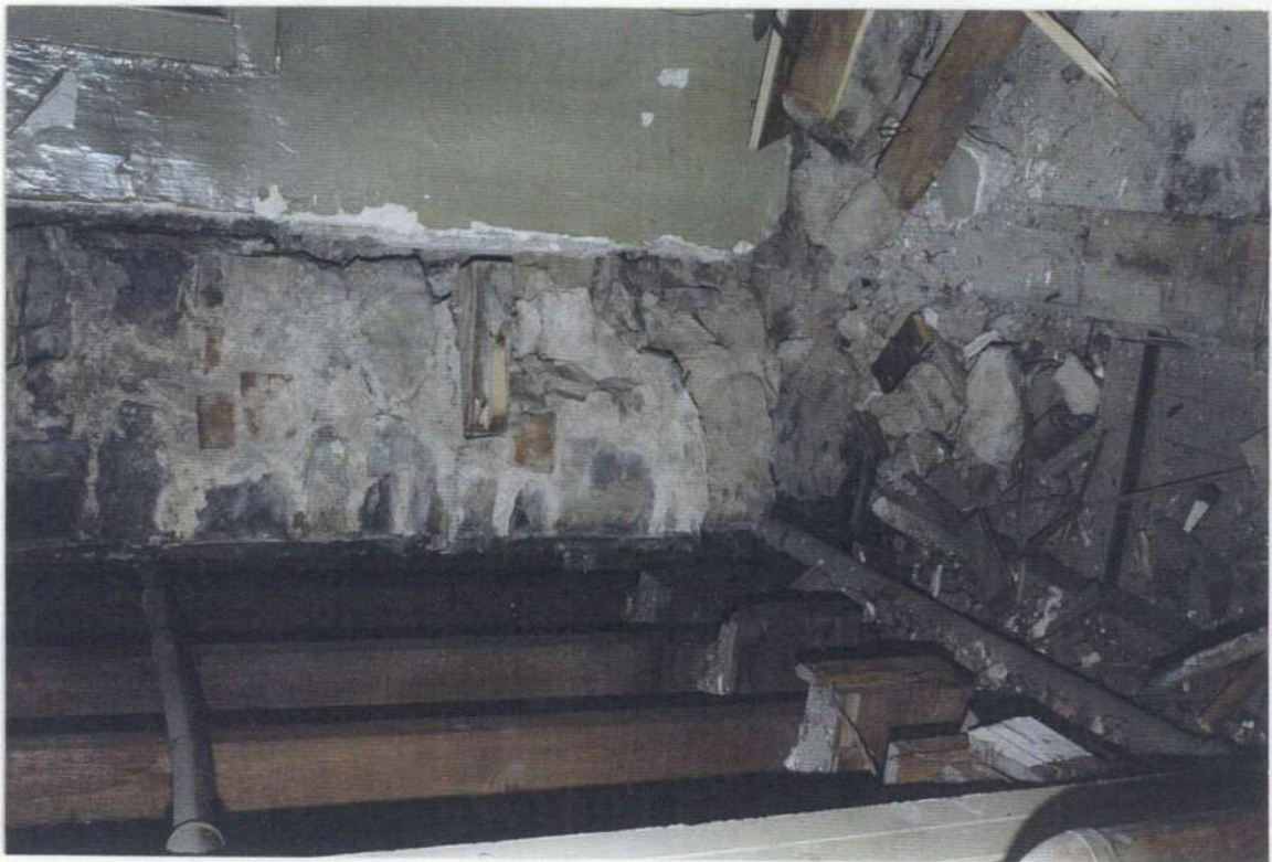
148l. Space 205. Southeast corner. Remains of stone wall removed in phase five. Note that edge of wide board planking stops at line of stone wall.
