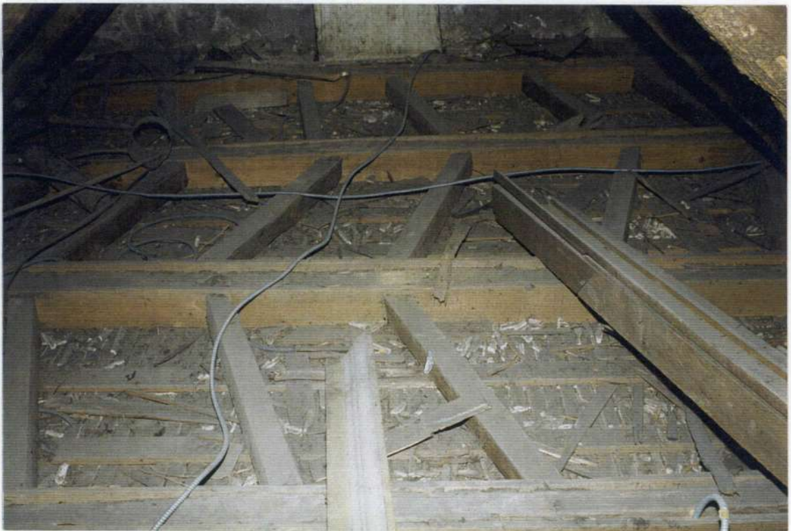
126. Second floor ceiling framing from attic.
