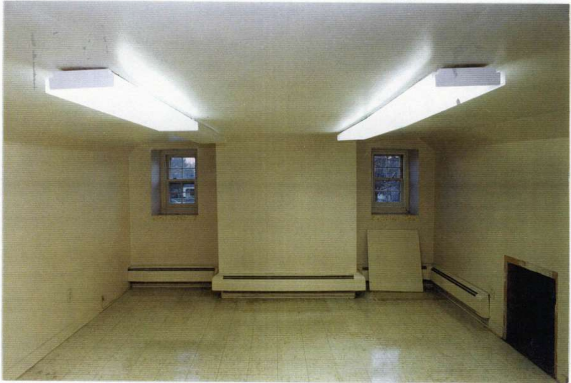
122. Space 204. South wall before removals.
