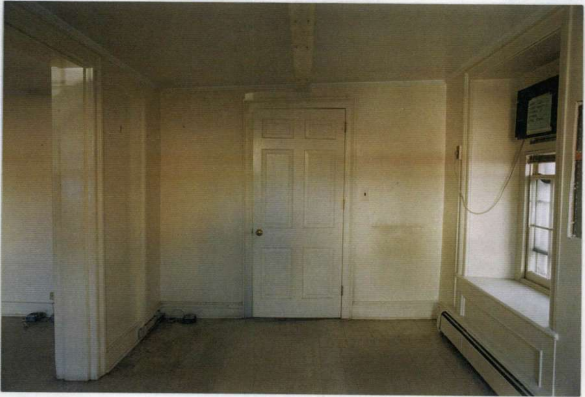
178. Space 108 west wall before removals.
