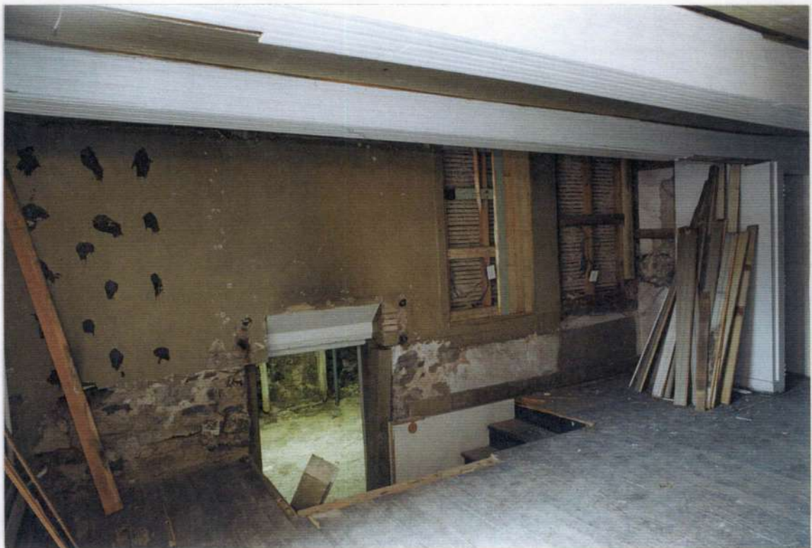
135. Space 104 west wall after removals. Note stone wall on south end and metal lath and plaster infill where stairs were removed.
