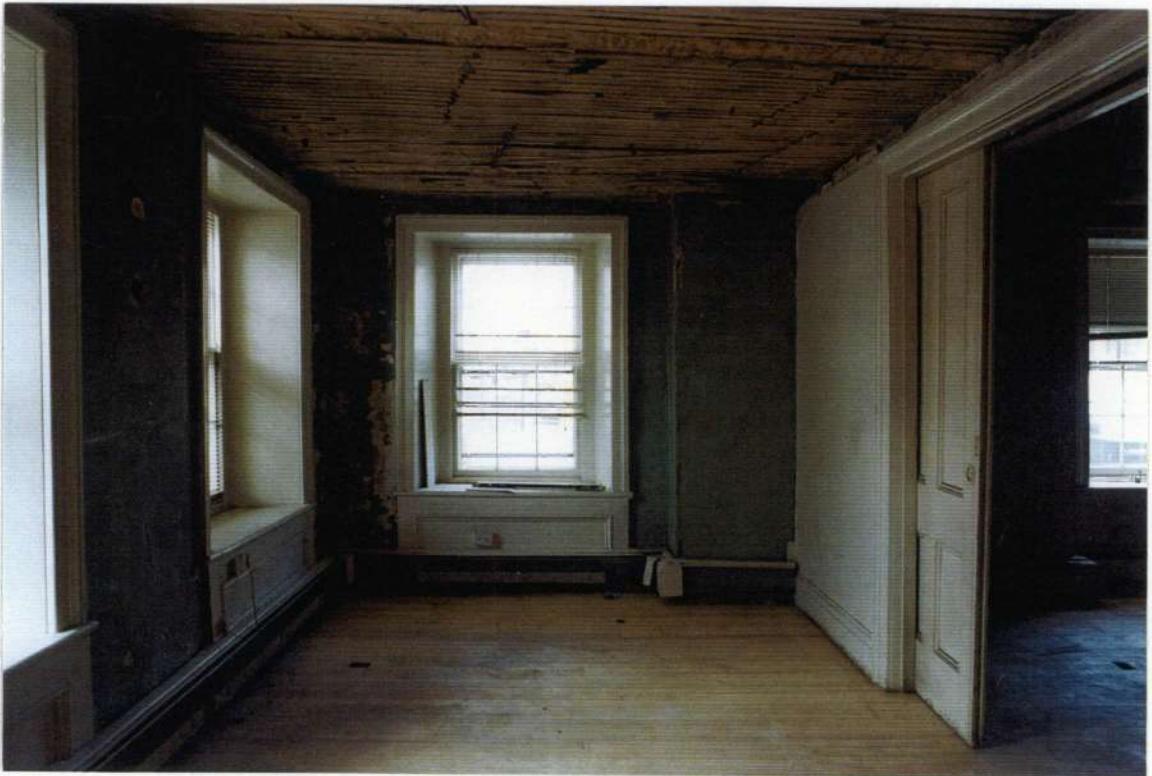
174. Space 108 east wall after removals. Note uncovered pocket doors.
