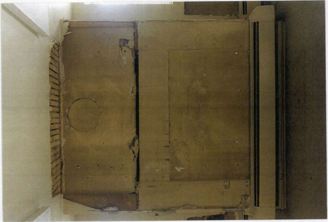
124. Detail: built-out chimney breast and mantel. Note round sheetmetal stove pipe connection.
