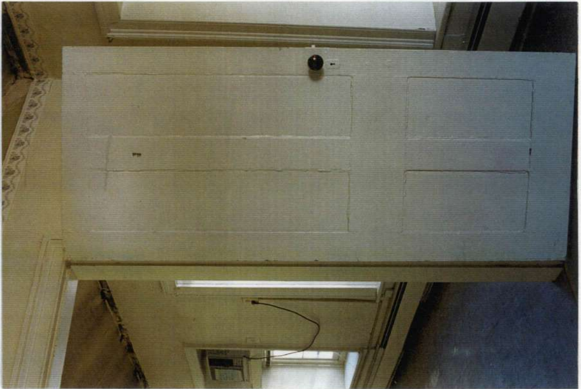
213. Door between space 206 and 207 as seen from 207.
