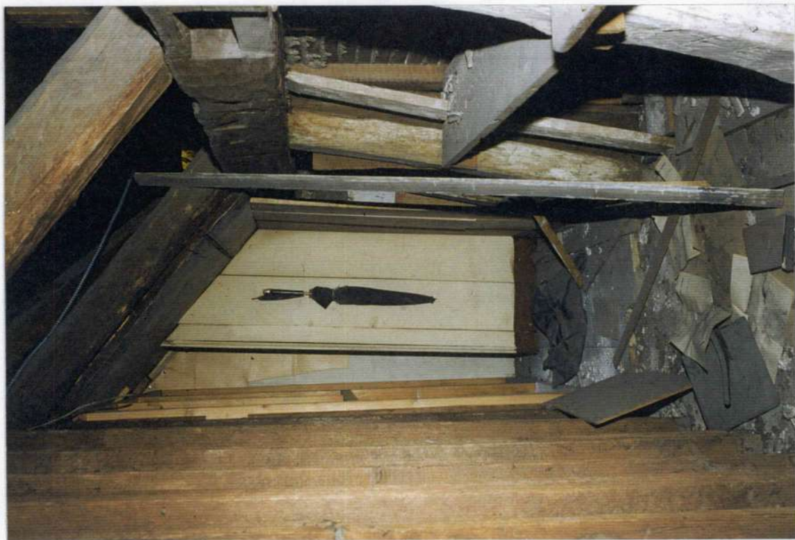
128. Space 204B looking north. Note that horizontal timber that supports the roof rafters has a mortise hole on the side, appears to be a recycled timber.
