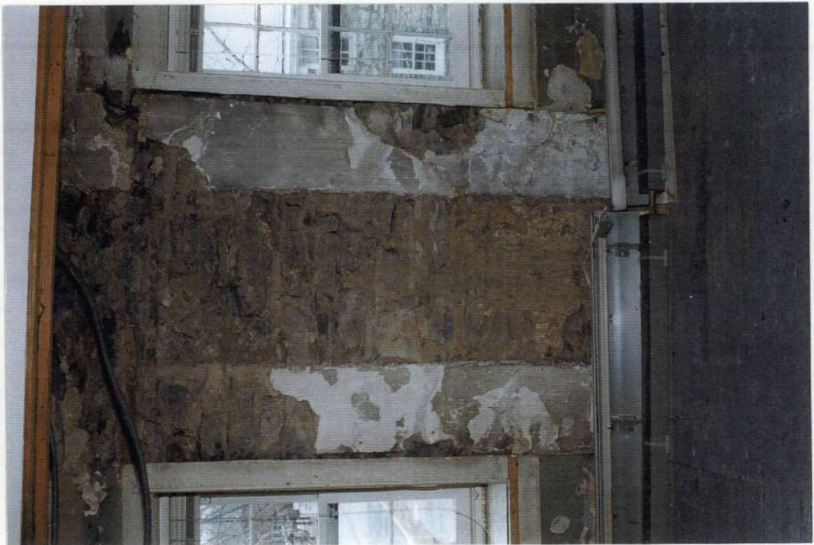
74. Detail: Shadow of removed chimney and chimney breast.
