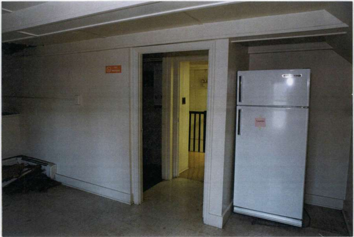
83. Space 201. South wall before removals.
