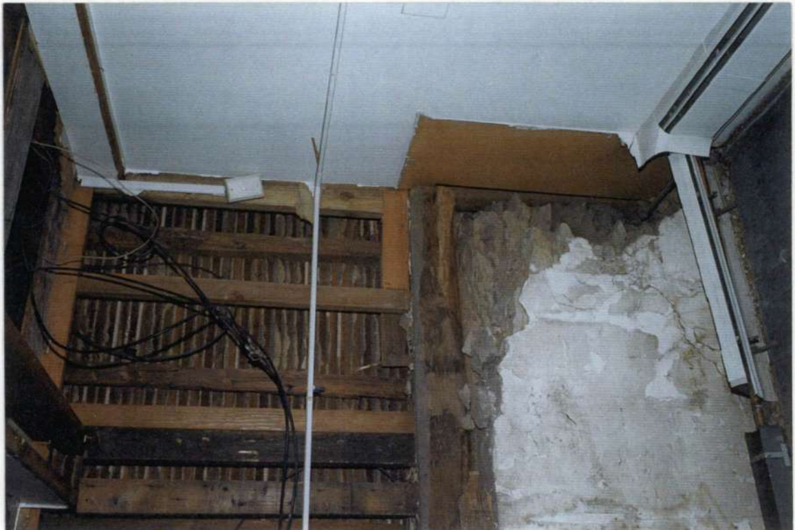
78. Detail: Removed stone wall on south end of east wall room 201.
