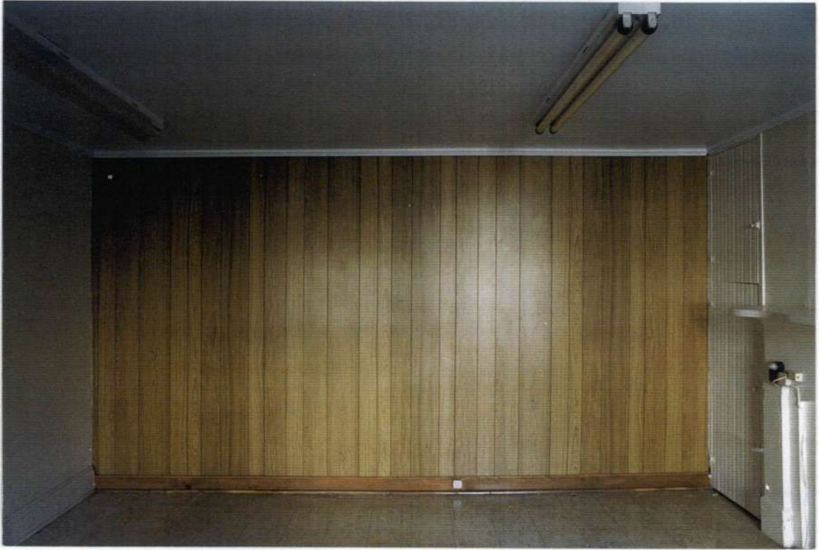
166. Space 105 south wall before removals.
