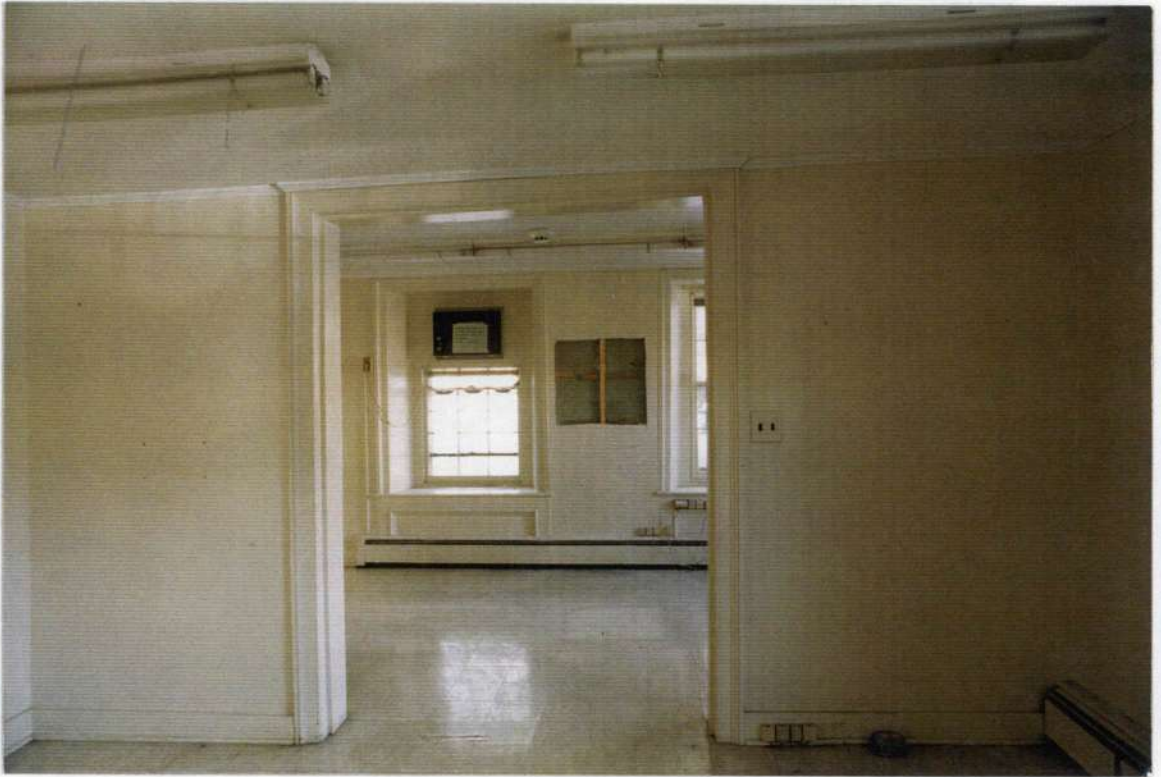
183. Space 109 north wall before removals.
