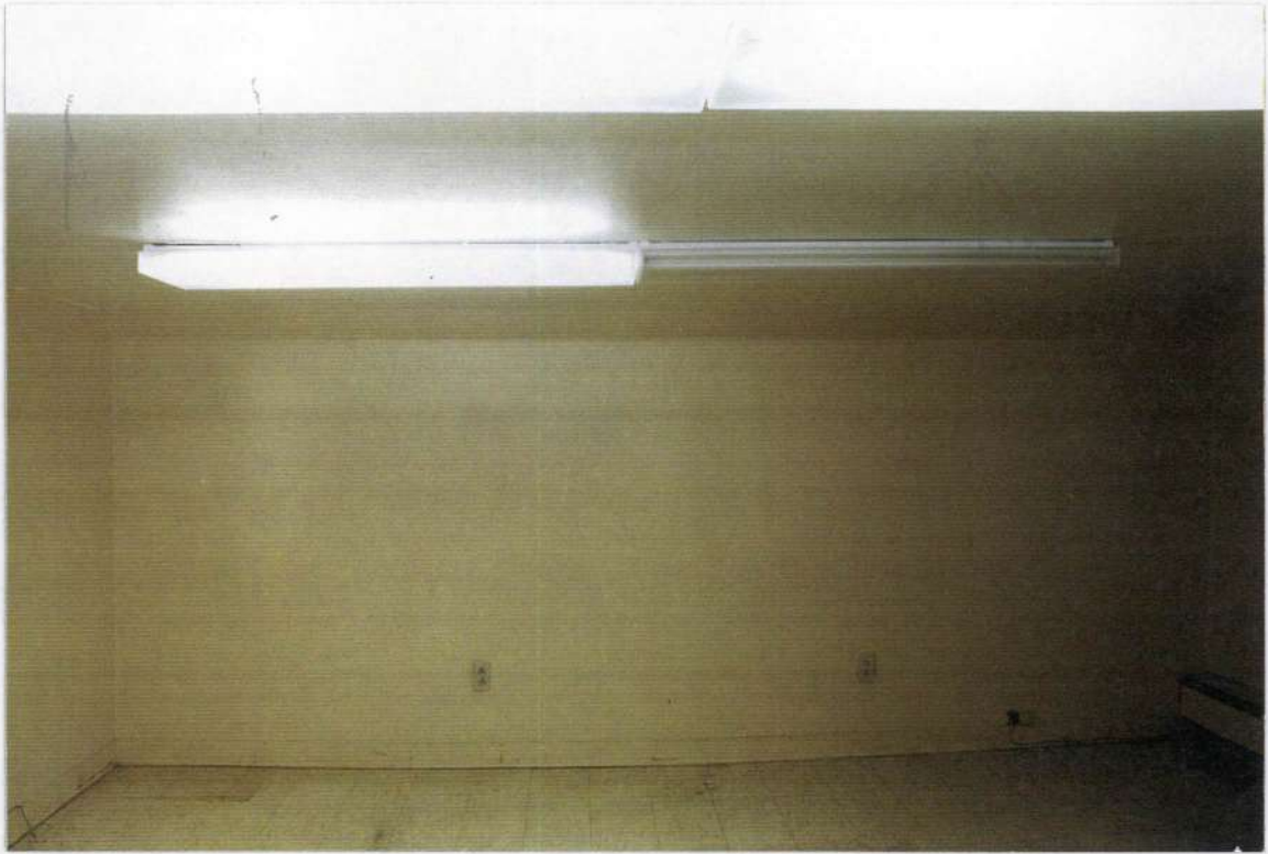
116. Space 204. East wall before removals.
