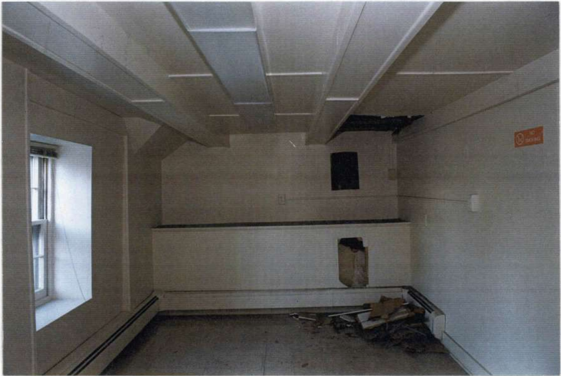
69. Space 201. East wall before removals.
