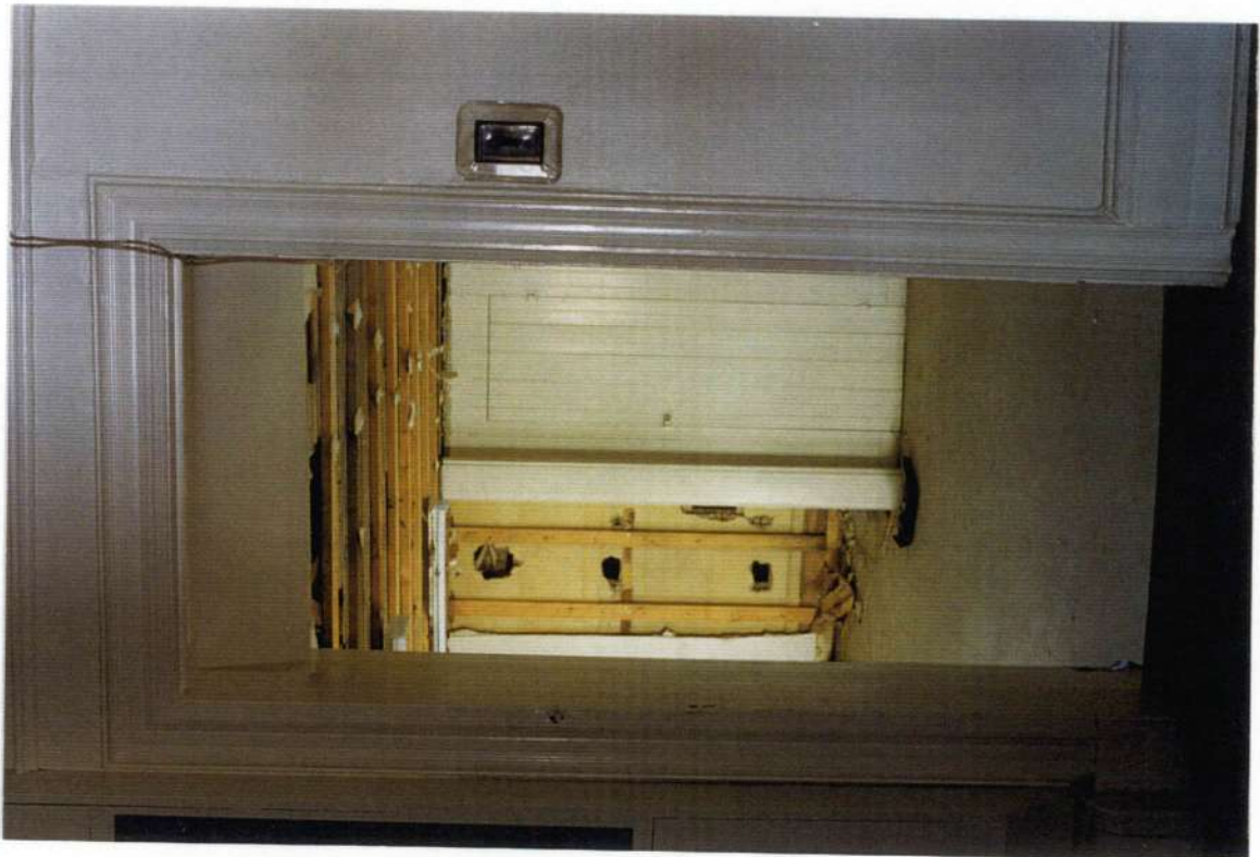
141a. Opening from space 211 into space 205.
