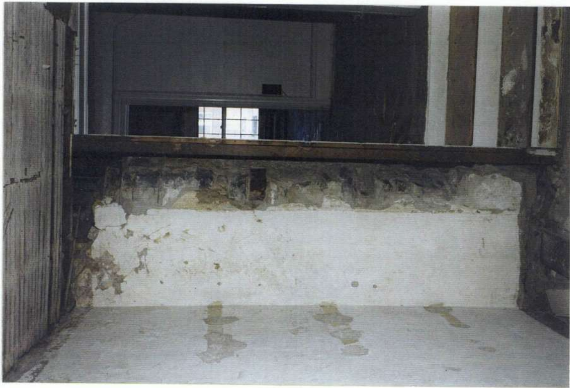
148h. Space 205 northeast corner of remains of phase four stone wall added to phase three east wall.
