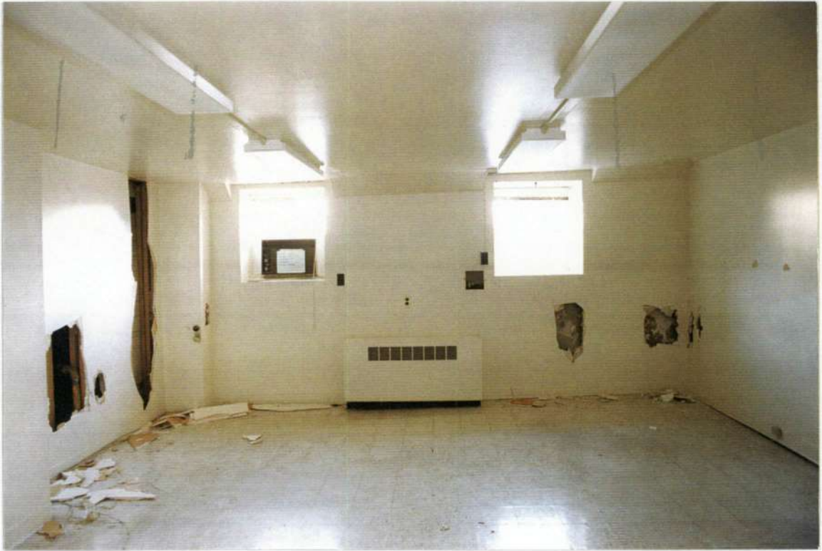
145. Space 205 south wall before removals.
