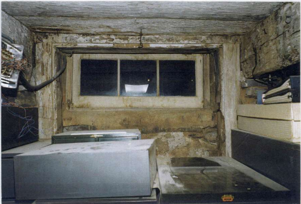
101. Detail: Mortise and tenon pegged door frame and later cellar window.
