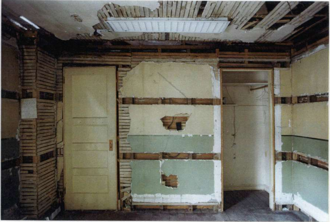
240. Space 212 south wall door to left was covered by recent paneling.
