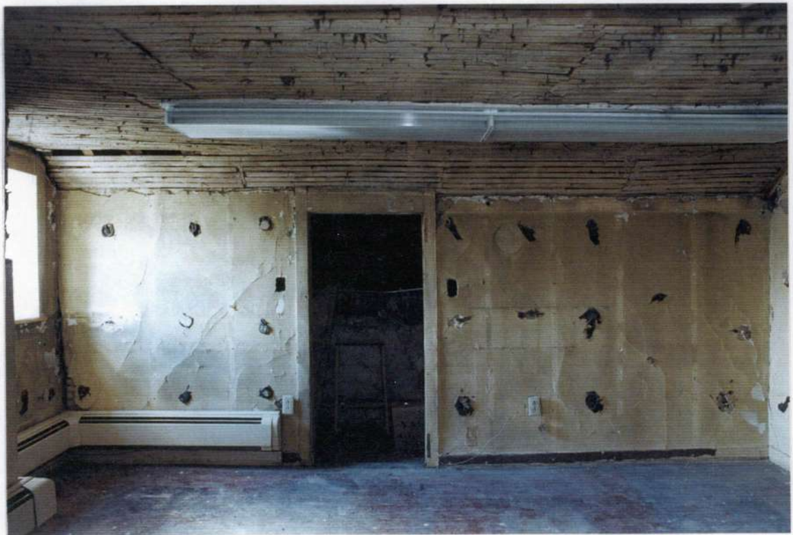
121. Space 204. West wall after removals. Note covered door frame.
