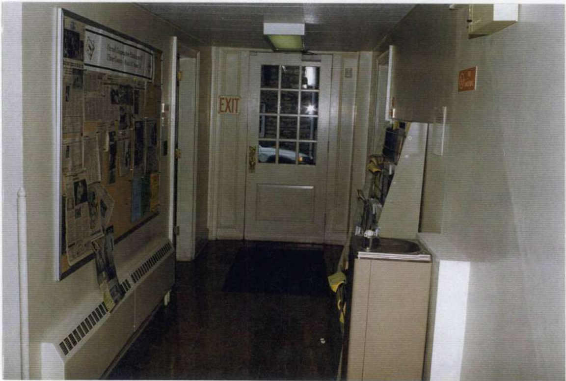
177a. Space 106. John Street entrance door looking north.
