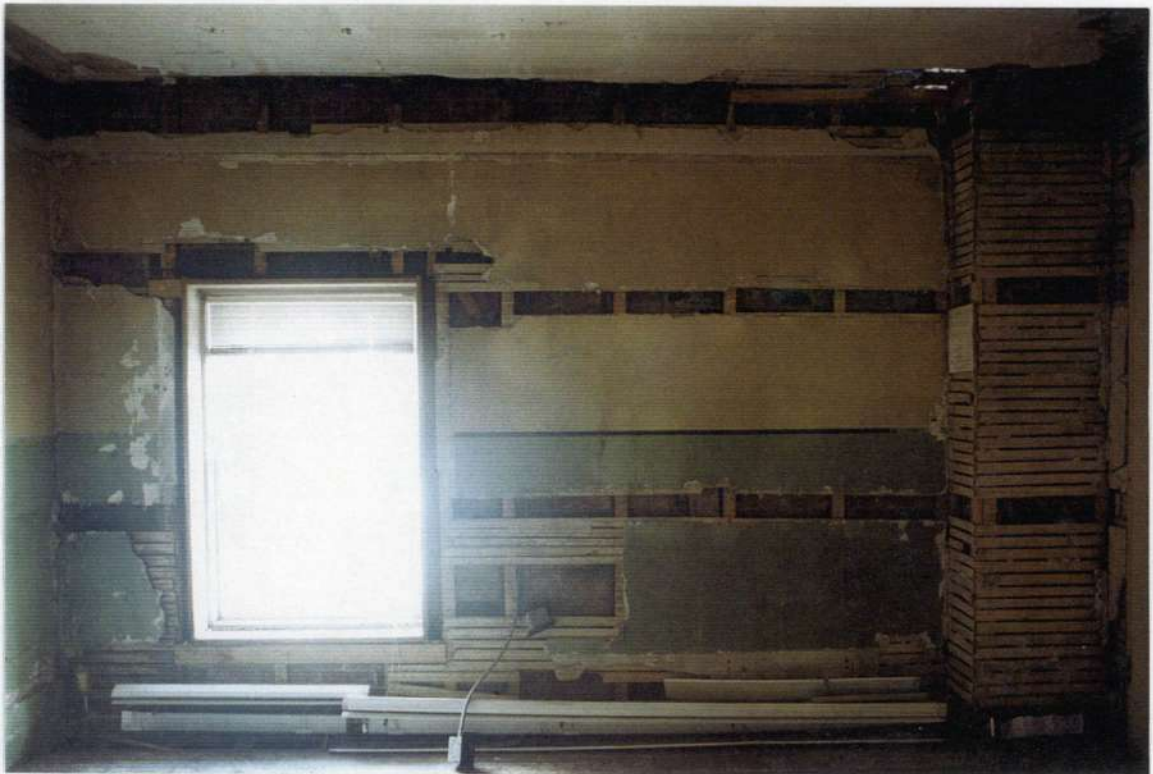
241. Space 212 east wall after removals.
