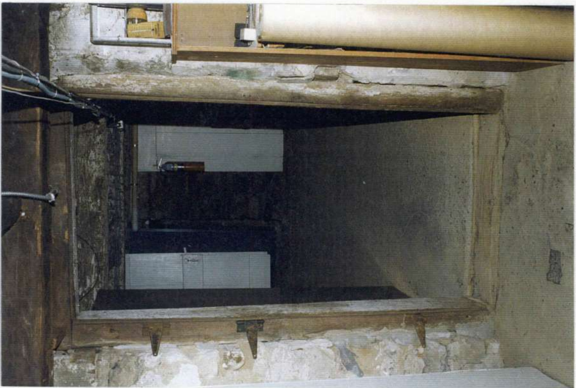
99. Detail: Heavy timber mortise and tenon pegged door frame between phase two and phase one as seen from space 001. Note possible pegged timber threshold at buried floor.
