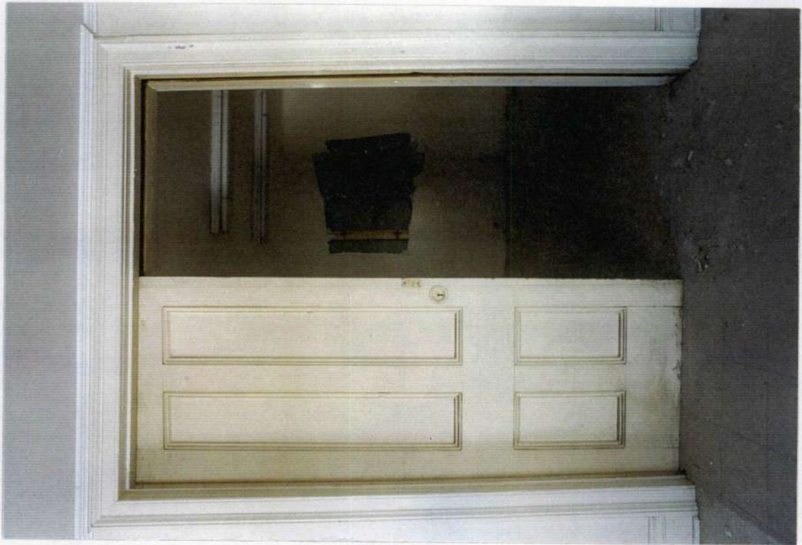
182. Detail: pocket doors in wall phase five.
