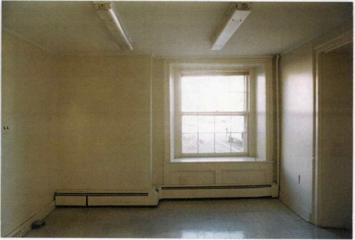
189. Space 109 east wall before removals.
