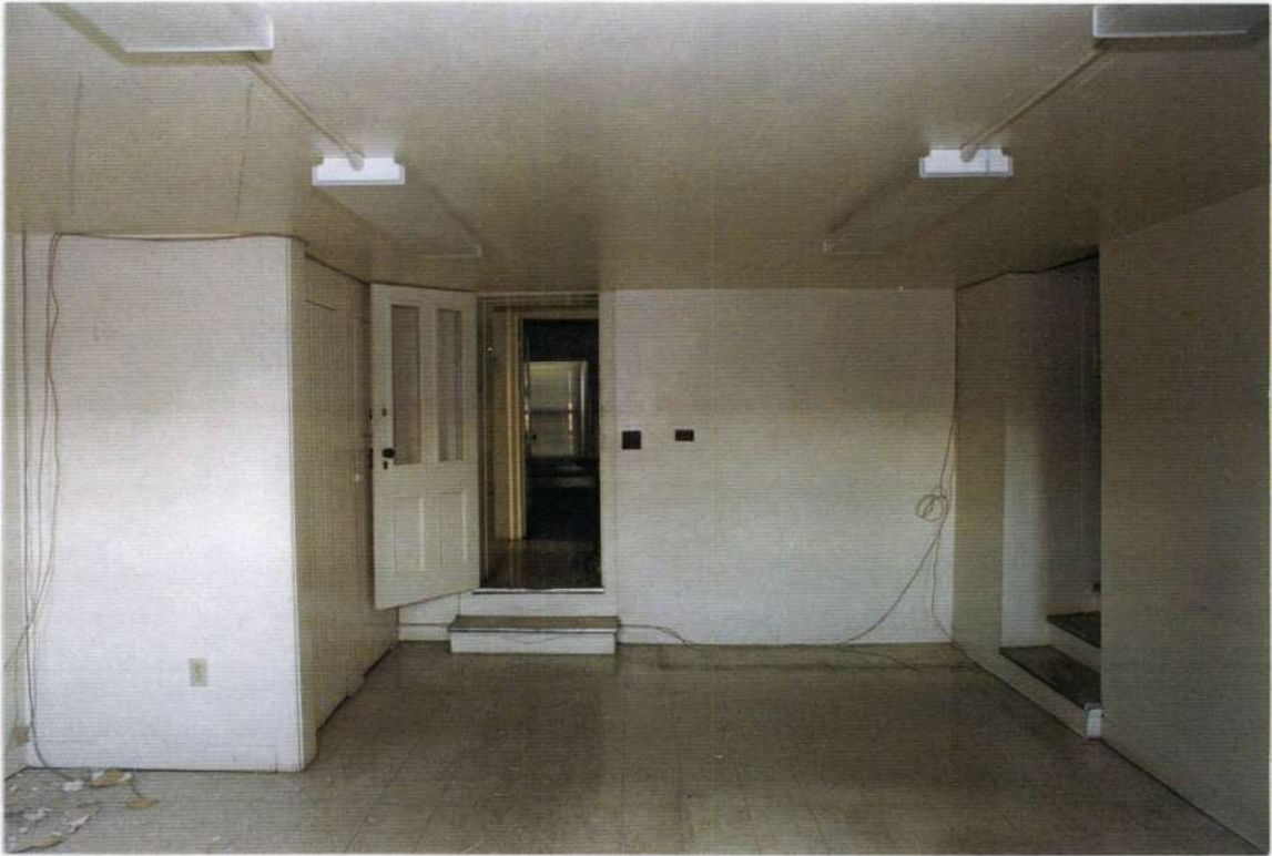
139. Space 205 north wall before removals.
