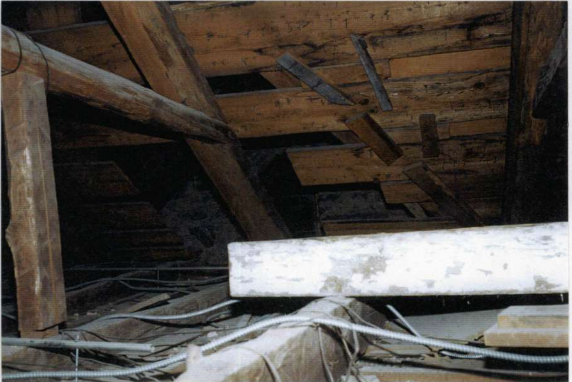
220. Attic over space 206 looking at ca. 1850s gable dormer.
