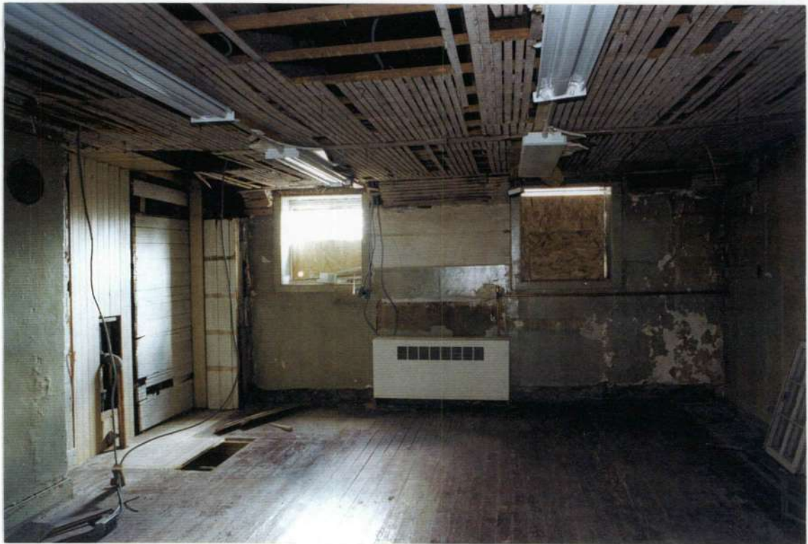
145. Space 205 south wall after removals.
