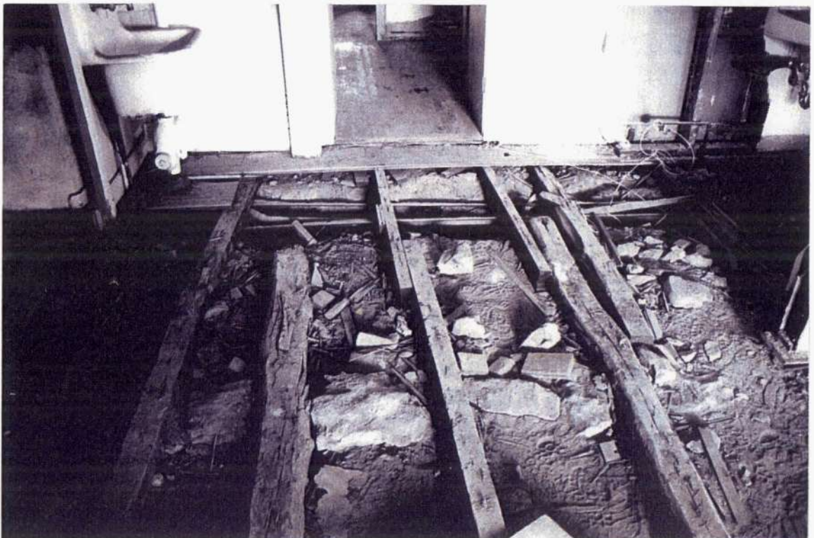
Photograph 5. Phase 3 with flooring removed. View North.
