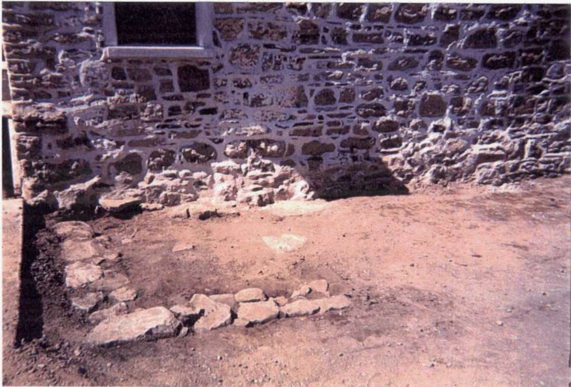
Photograph 28. South yard looking at Phase 2/3 wall. View North.
