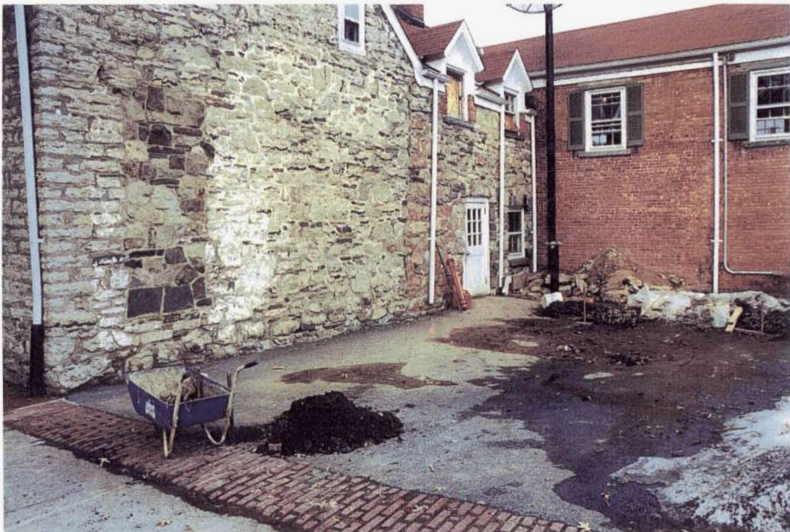
Photograph 26. South yard showing shovel testing through macadam. View NE.
